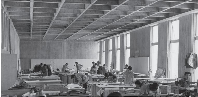
**Figure 4.** Learning Laboratory: Radial Reinforced concrete beams, waffle slabs.
