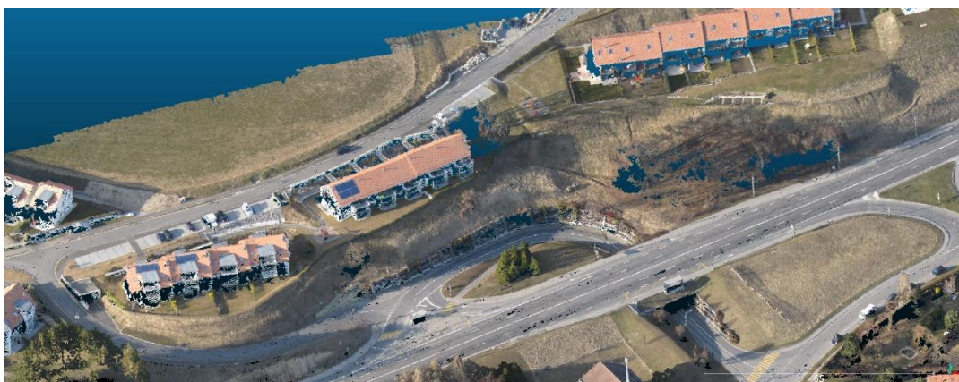
Figure 100: Steep slope example with complex road structure
