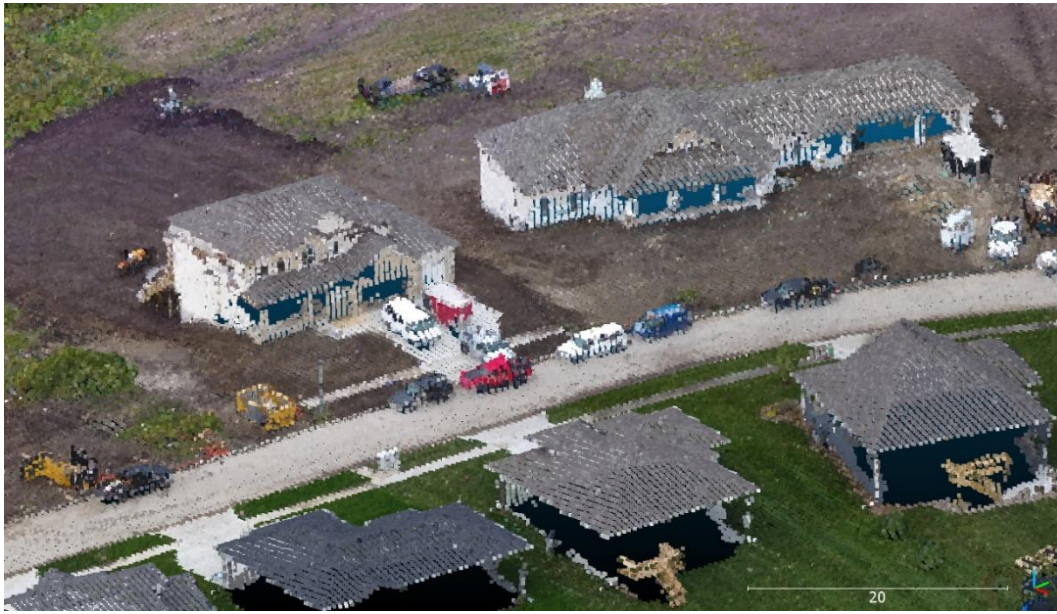
Figure 94: Vehicles and other objects before removal
