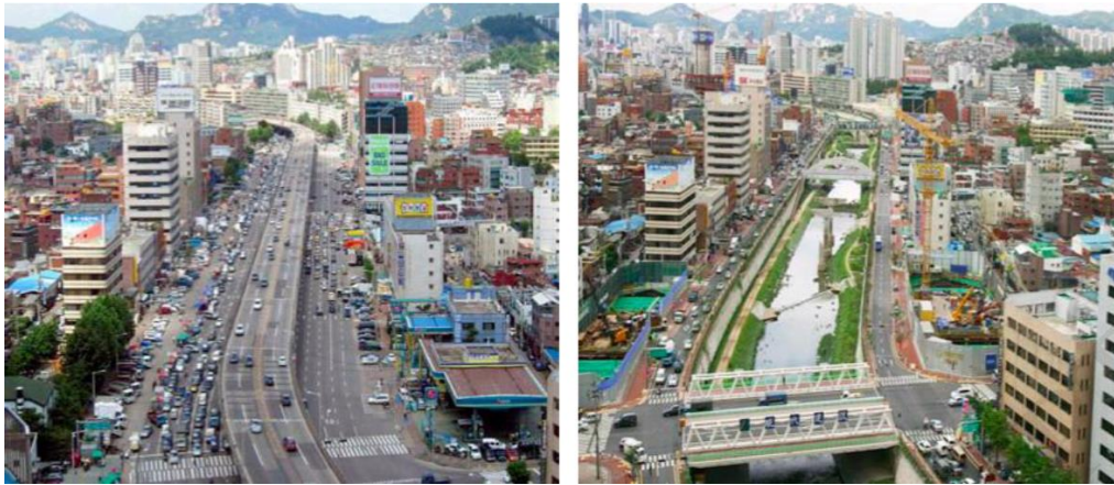
Figure 3.9. Before and after the daylighting project in Seoul (Kim & Jung, 2018).
