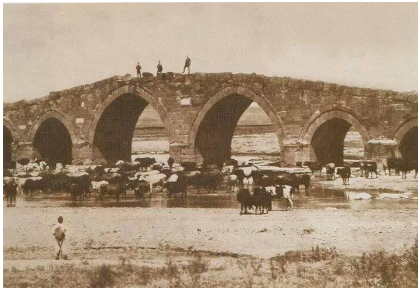
Figure 4.18. Akköprü Bridge 1917. The animals drink water.
