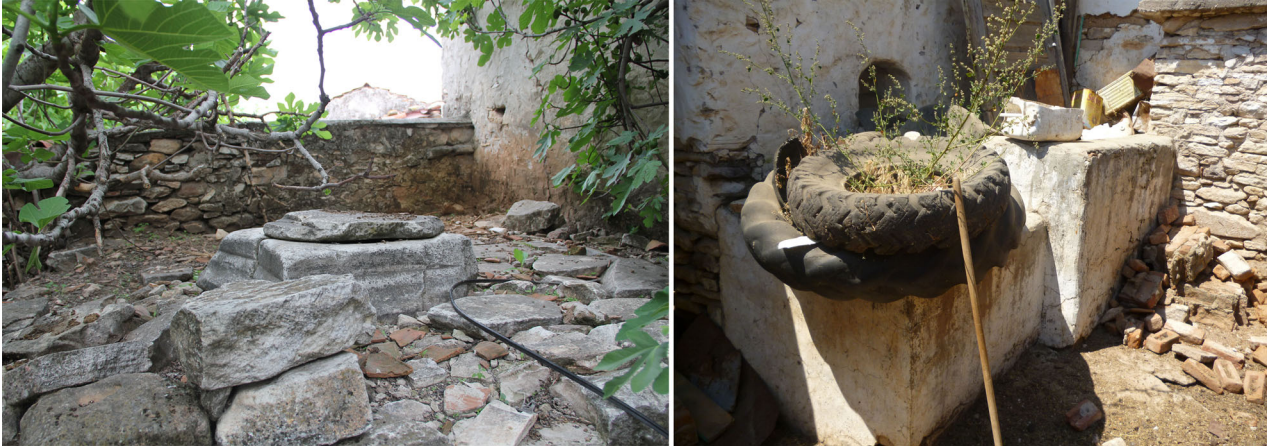
Figure 10. A well to store rainwater in the courtyard of a house (left) and an apilimi attached to the courtyard wall of another house (right).
