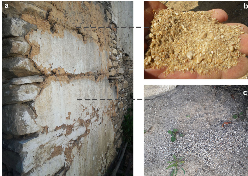
Figure 24. (a) Double-layer plaster on the wall, (b) yellow soil for the mud plaster, (c) fine sand for the lime plaster.
