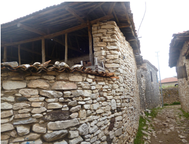
Figure 23. Roads bordered with thick stone masonry walls of the houses and courtyards.
