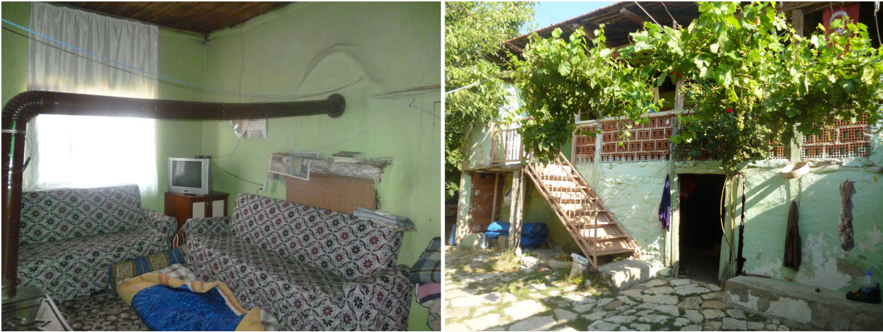
Figure 27. Closed fireplace in a room (left) and steel staircase addition in the courtyard (right).
