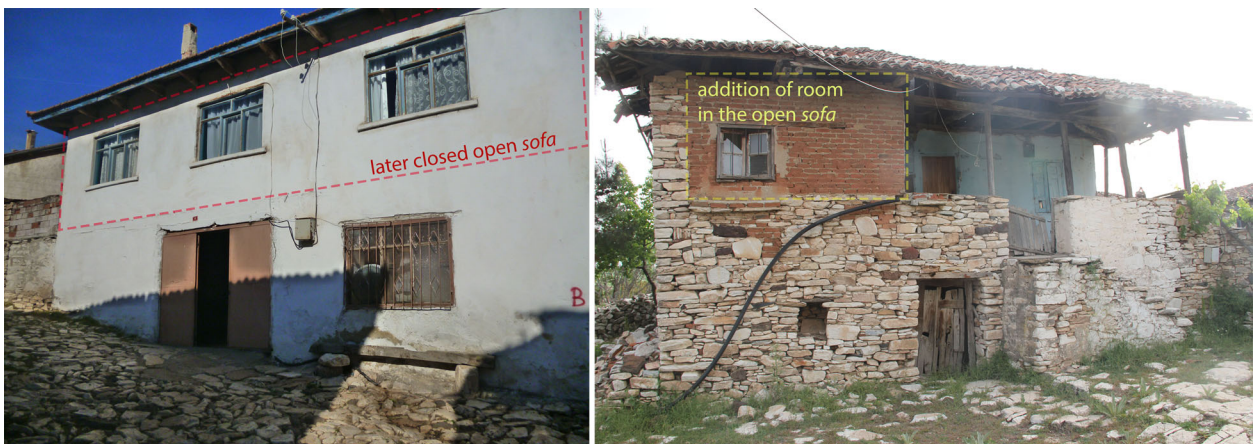
Figure 26. A house where the outer sofa was later closed (left) and the addition of a room in the outer sofa of another house (right).
