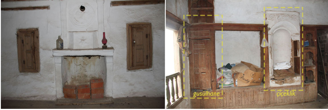
Figure 21. Fireplace with two embedded cupboards (left); gusülhane and çiçeklik in wooden cupboard in the room of a house located in the Rum neighbourhood (right).
