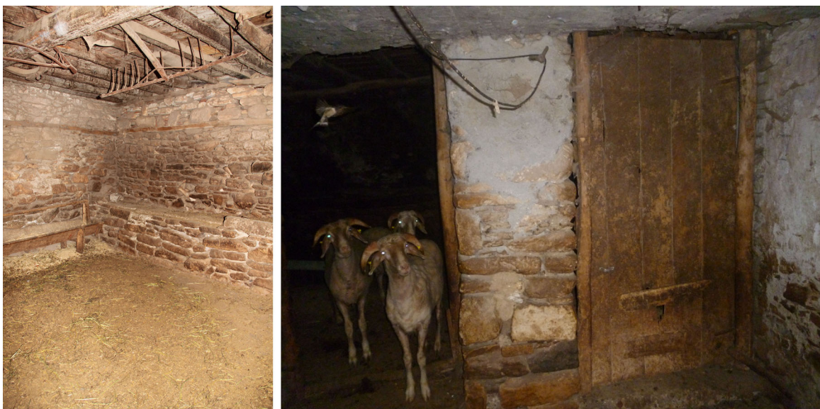
Figure 12. Stable of a house and the low stone masonry platform (tabla), on one side of the stable.
