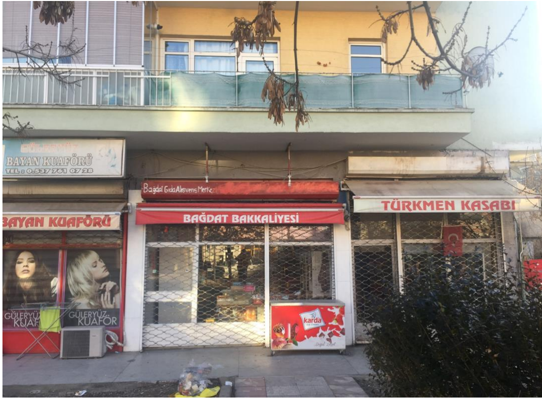
Figure 18 Façades of the Türkmen shops. Photo by the author. 9 October 2020.
