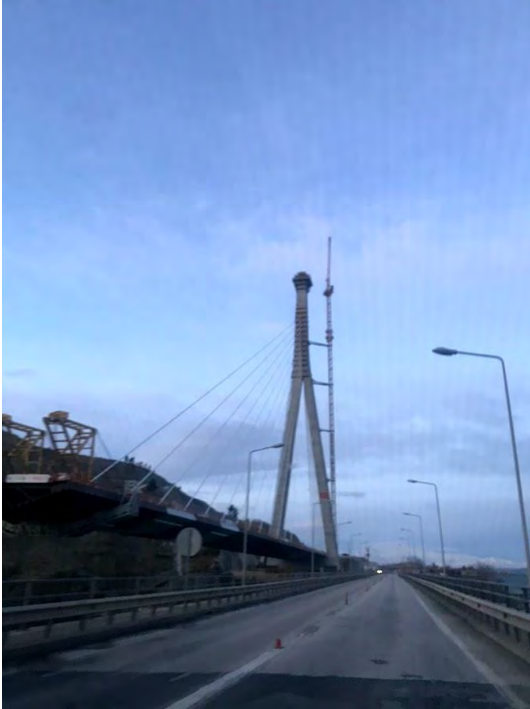
Figure 4.60. New K m rhan Bridge under construction on Fırat River (38°26'29.6"N 38°49'10.3"E / 01.02.2020 / 7:25)
