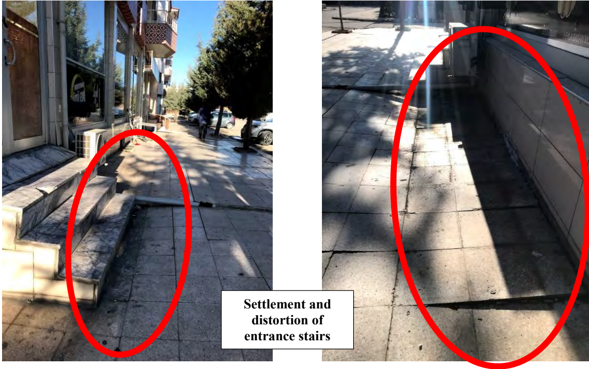
Figure 4.104. Settlements observed ( 38^{\circ}40'05.7''N 39^{\circ}11'09.6''E / 01.02.2020 / 15:57 & 38^{\circ}40'05.1''N 39^{\circ}11'10.0''E / 01.02.2020 / 15:57)
