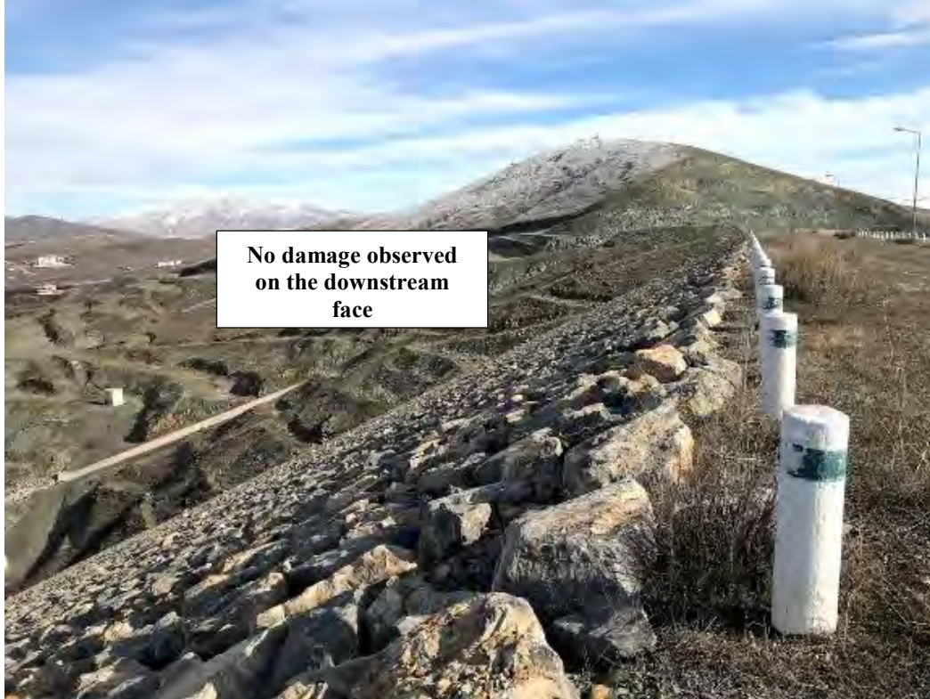
Figure 4.76. Side view of Kapıkaya Dam downstream face ( 38^{\circ}21'16.3''N 38^{\circ}36'33.2''E / 01.02.2020 / 10:40 & 38^{\circ}21'13.1''N 38^{\circ}36'26.7''E / 01.02.2020 / 10:46)
