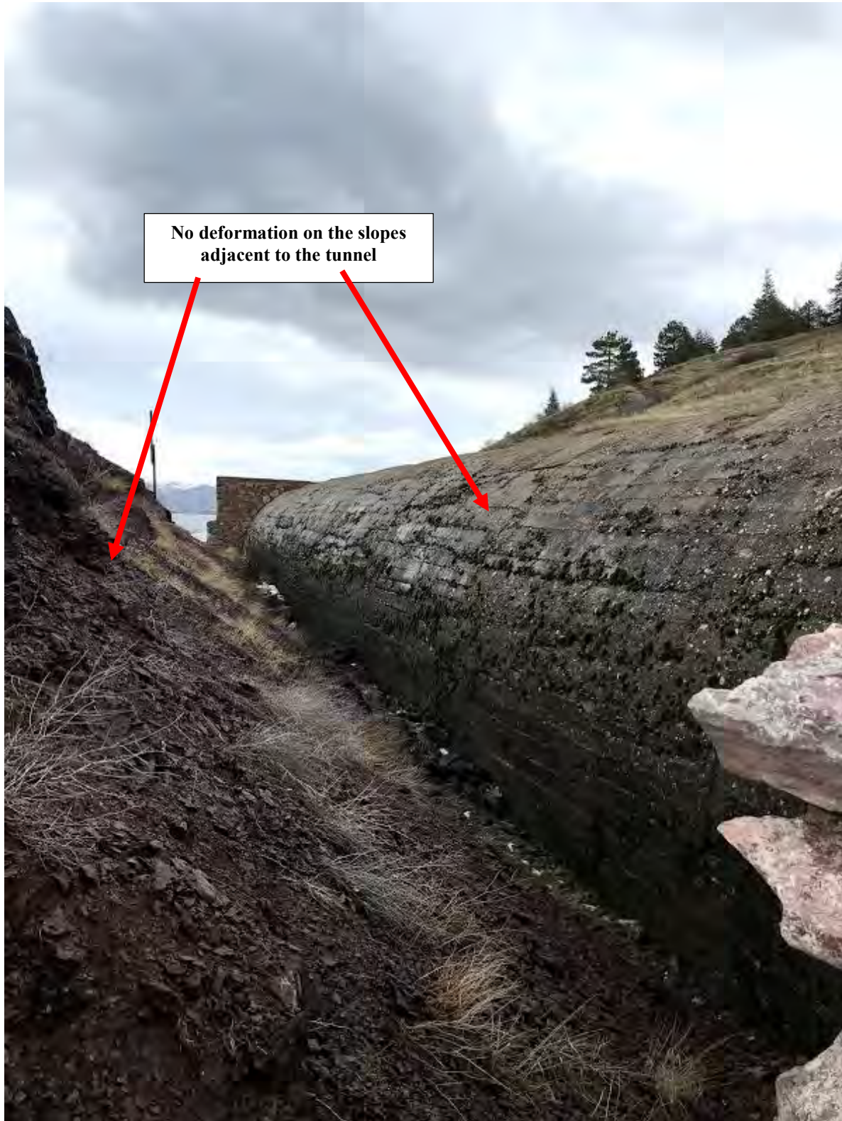
Figure 4.41. A view of tunnel body at Stop 10 ( 38^{\circ}28'53.2''N 39^{\circ}27'18.4''E / 31.01.2020 / 15:09)
