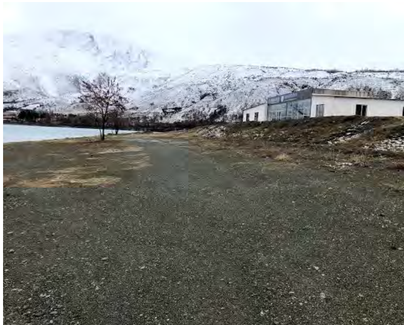
Figure 4.21. No ground failure on a neighboring beach of Hazar Lake ( 38^{\circ}26'48.9''N 39^{\circ}18'59.4''E / 31.01.2020 / 13:08)
