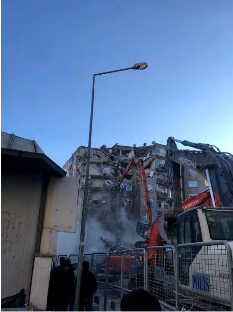
Figure 4.110. Demolishment of a heavily-damaged building in the Mustafa Paşa district of Elazığ city center (38°40'15.2"N 39°13'57.5"E / 01.02.2020 / 16:31)
