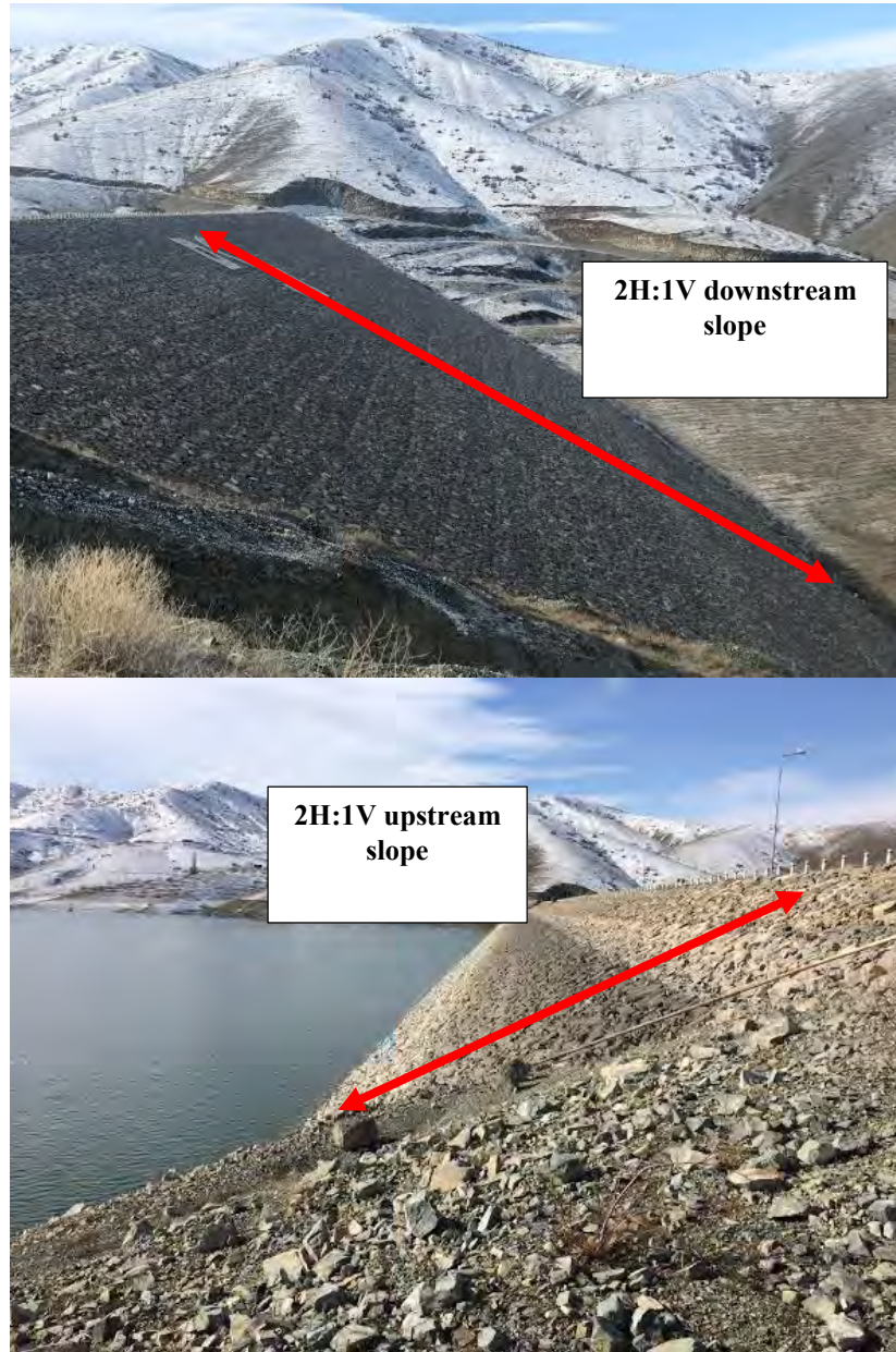
Figure 4.75. Side views of Kapıkaya Dam (38°21'19.1"N 38°36'33.9"E / 01.02.2020 / 10:21 & 38°21'16.3"N 38°36'35.0"E / 01.02.2020 / 10:38)
