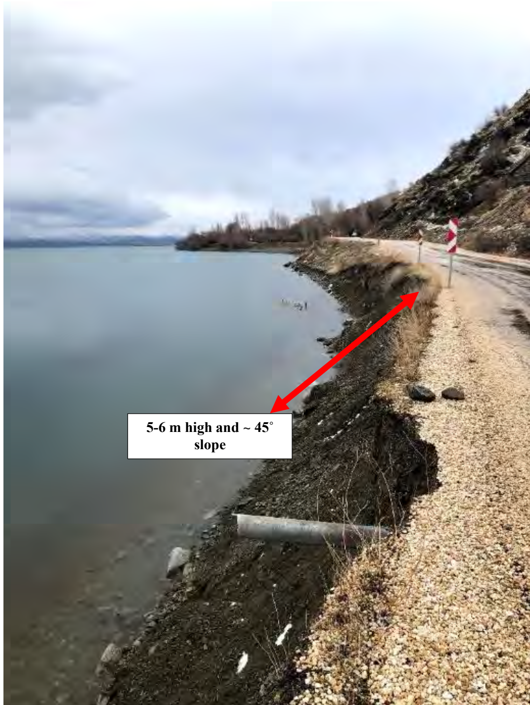
Figure 4.29. No failure on the road embankment ( 38^\circ 26' 43.7'' N 39^\circ 20' 40.7'' E / 31.01.2020 / 13:54)
