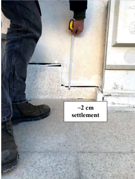
Figure 4.103. Settlement mapped at the entrance of some buildings ( 38^{\circ}40'04.7''N 39^{\circ}11'12.4''E / 01.02.2020 / 15:31 & 38^{\circ}40'05.9''N 39^{\circ}11'08.2''E / 01.02.2020 / 15:41 38^{\circ}40'05.9''N 39^{\circ}11'08.1''E / 01.02.2020 / 15:41 & 38^{\circ}40'04.7''N 39^{\circ}11'09.7''E / 01.02.2020 / 15:40)
