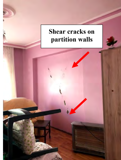
Figure 4.106. Cracks on partition walls ( 38^{\circ}40'03.9''N 39^{\circ}11'13.5''E / 01.02.2020 / 15:35 & 38^{\circ}40'04.2''N 39^{\circ}11'14.2''E / 01.02.2020 / 15:36)
