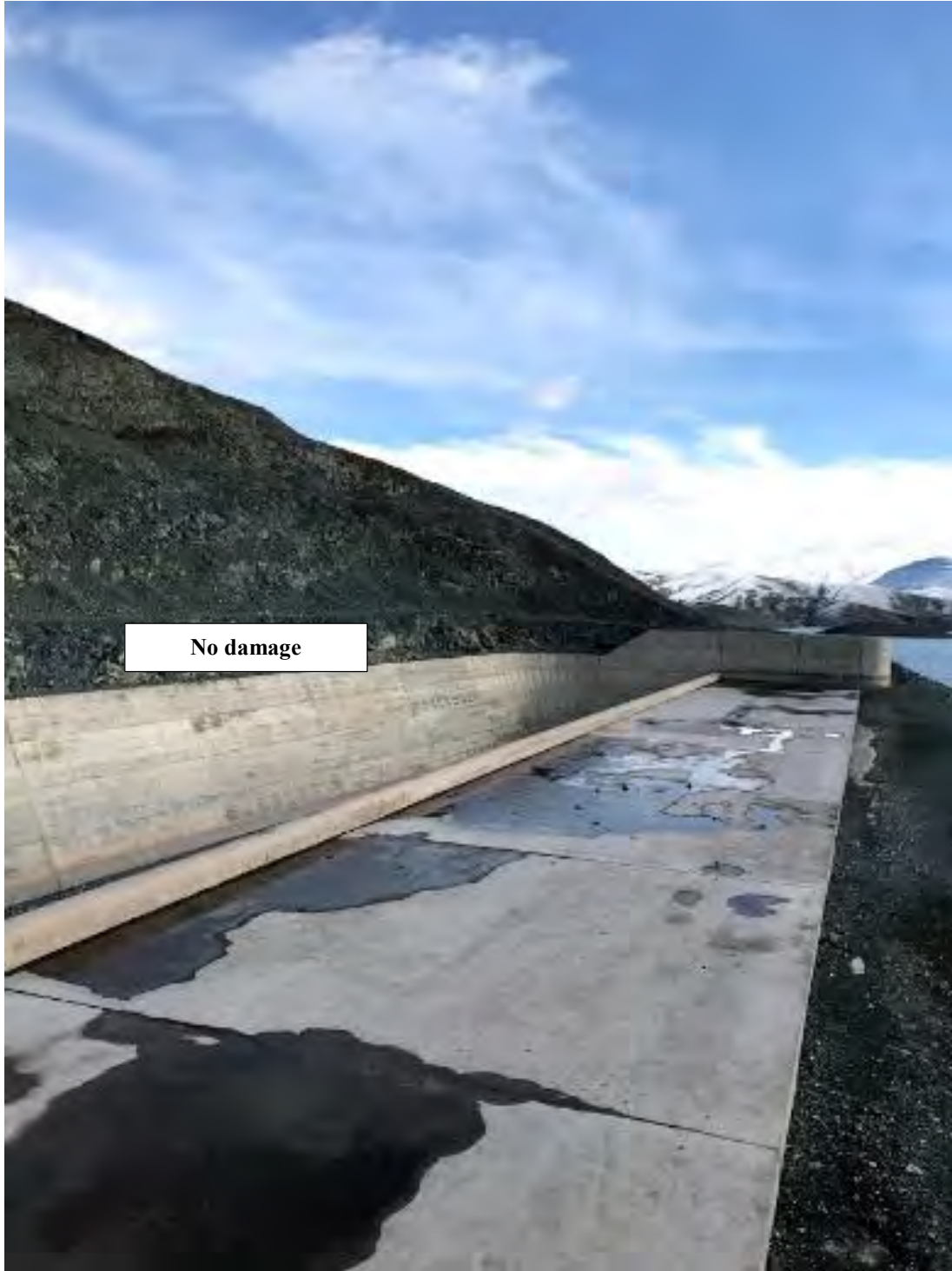
Figure 4.78. Water in-take structure of Kapıkaya Dam ( 38^{\circ}21'16.9''N 38^{\circ}36'36.0''E / 01.02.2020 / 11:13)
