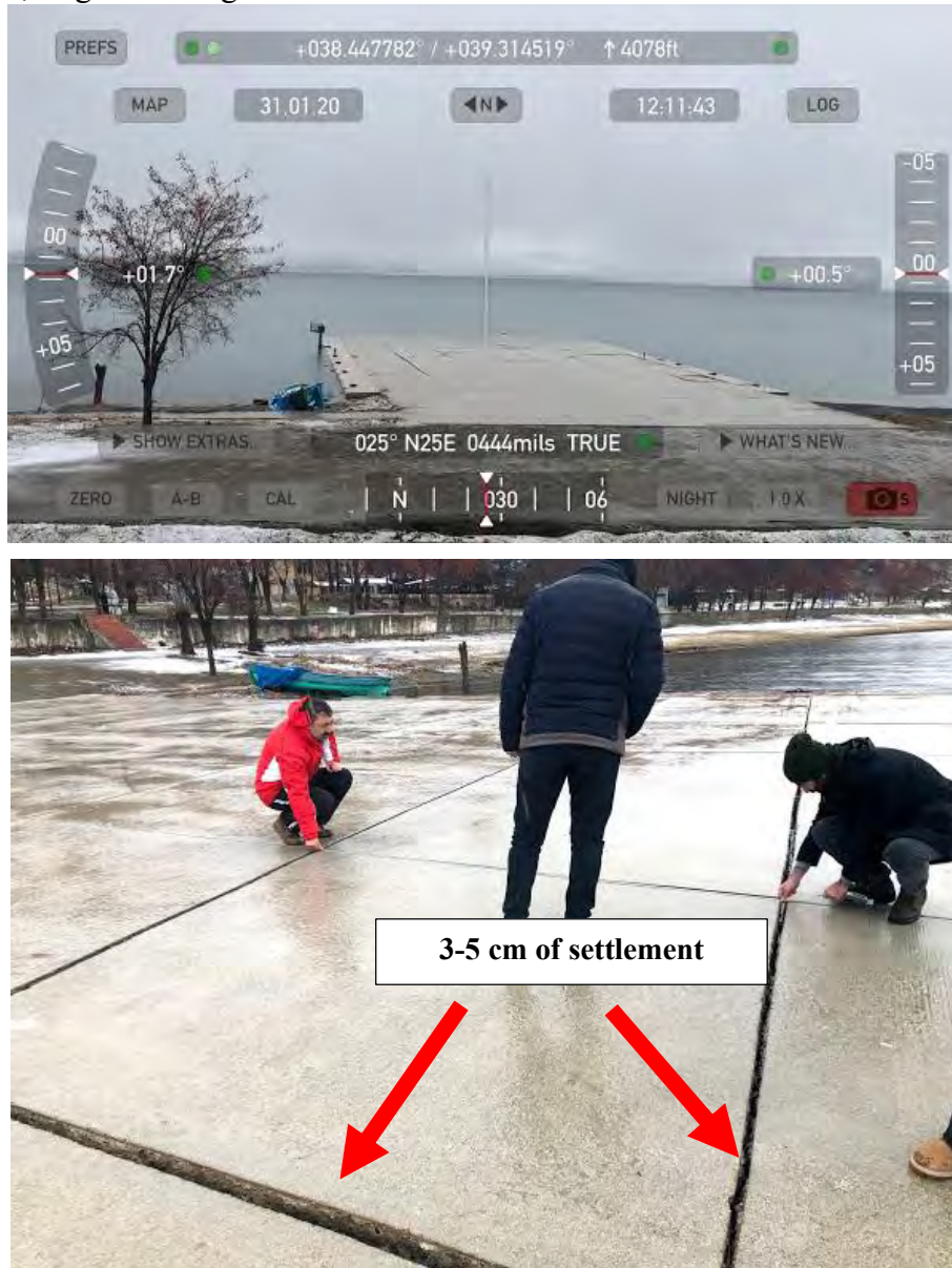
Figure 4.12. Seismically-induced volumetric settlement in the dock of Hazar Lake (38°28'10.0"N 39°17'03.6"E / 31.01.2020 / 12:11 & 38°26'53.2"N 39°18'53.4"E / 31.01.2020 / 12:14)
