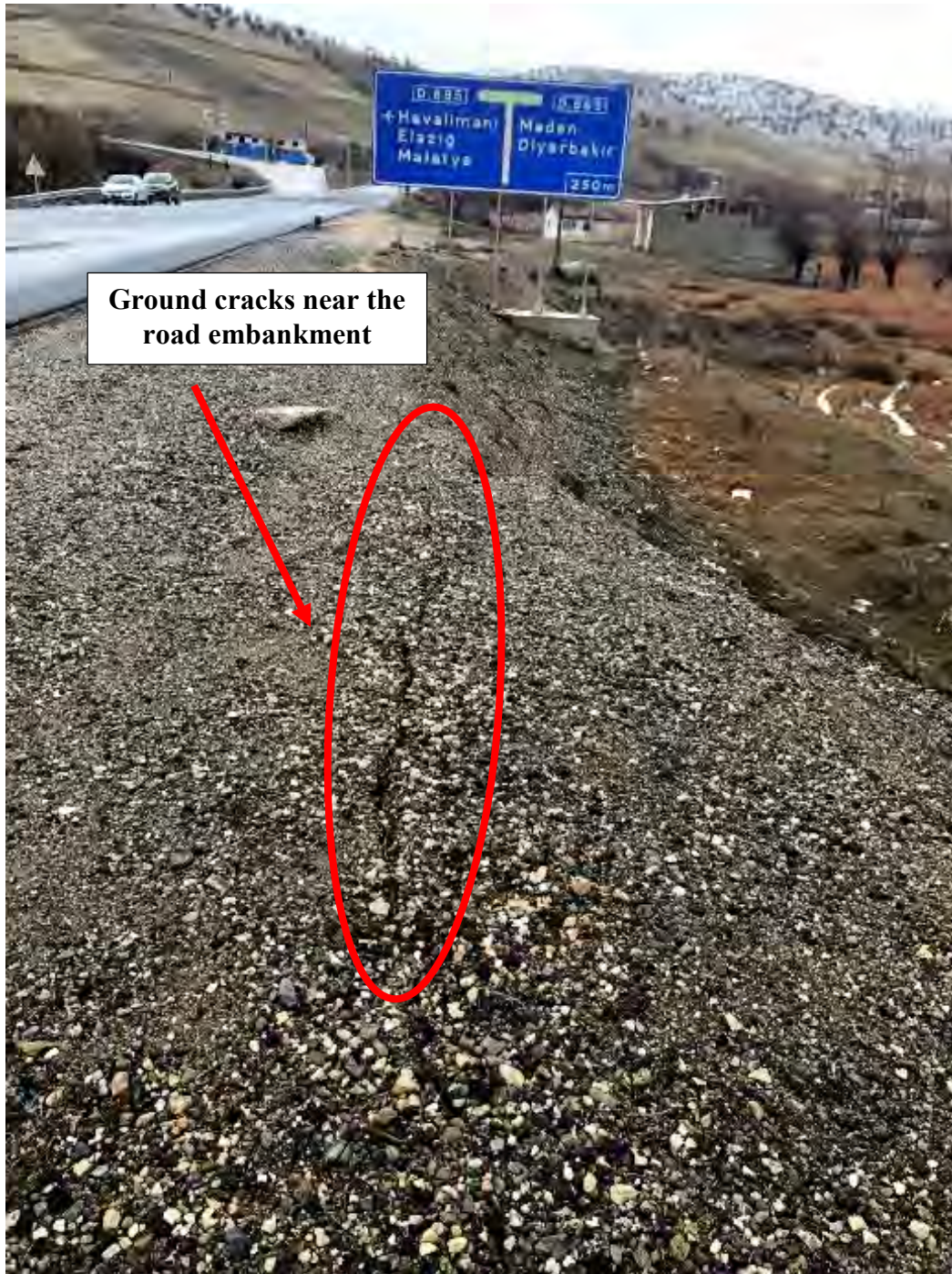
Figure 4.9. A small crack observed near the highway embankment ( 38^{\circ}28'08.0''N 39^{\circ}16'38.7''E / 31.01.2020 / 11:50)
