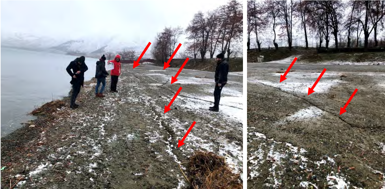
Figure 4.124. Deformations and cracks due to lateral spreading observed along Hazar Lake (2 nd stop)
