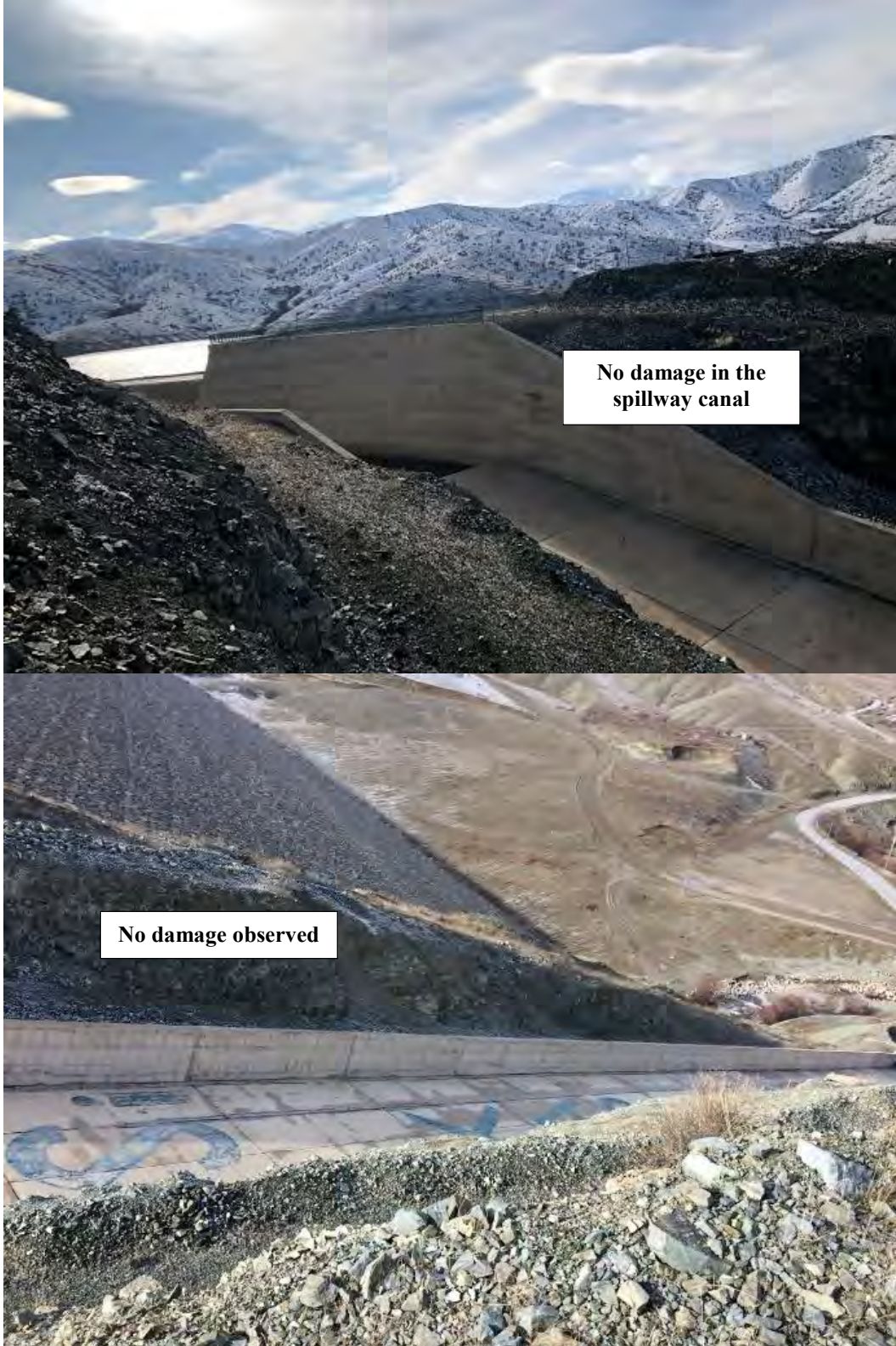
Figure 4.80. Spillway of Kapıkaya Dam ( 38^{\circ}21'19.1''N 38^{\circ}36'33.9''E / 01.02.2020 / 10:22 & 38^{\circ}21'19.2''N 38^{\circ}36'34.1''E / 01.02.2020 / 10:22)
