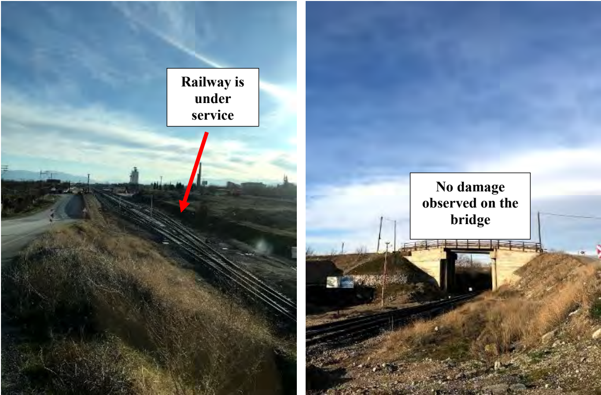
Figure 4.67. Railway and bridge at 20 th stop (38°26'00.1"N 38°21'59.1"E / 01.02.2020 / 8:49 & 38°26'00.2"N 38°22'01.3"E / 01.02.2020 / 8:50)
