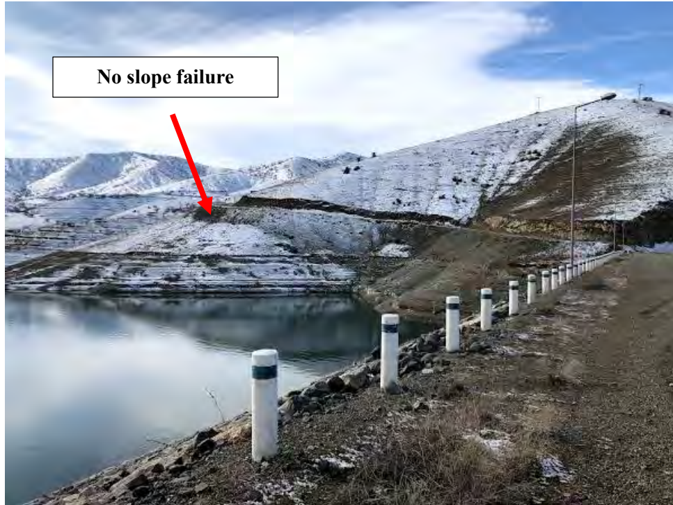
Figure 4.81. Abutment slopes of Kapıkaya Dam ( 38^{\circ}21'07.1''N 38^{\circ}36'22.0''E / 01.02.2020 / 10:51)
