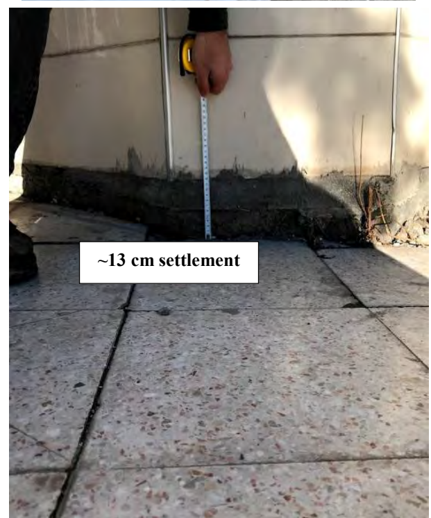
Figure 4.103. Settlement mapped at the entrance of some buildings ( 38^{\circ}40'04.7''N 39^{\circ}11'12.4''E / 01.02.2020 / 15:31 & 38^{\circ}40'05.9''N 39^{\circ}11'08.2''E / 01.02.2020 / 15:41 38^{\circ}40'05.9''N 39^{\circ}11'08.1''E / 01.02.2020 / 15:41 & 38^{\circ}40'04.7''N 39^{\circ}11'09.7''E / 01.02.2020 / 15:40)
