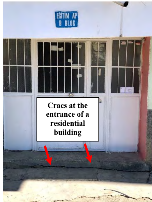
Figure 4.96. Cracks observed at the entrance of Eğitim Apartment. ( 38^{\circ}39'29.2''N 39^{\circ}09'01.6''E / 01.02.2020 / 14:31 & 38^{\circ}39'32.0''N 39^{\circ}09'00.8''E / 01.02.2020 / 14:36)
