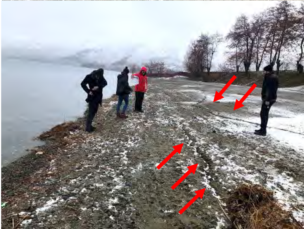
Figure 4.15. Seismically-induced lateral spreading on the beach of Hazar Lake ( 38^{\circ}26'53.7''N 39^{\circ}18'54.2''E / 31.01.2020 / 12:21 & 38^{\circ}26'50.7''N 39^{\circ}18'56.9''E / 31.01.2020 / 12:21)
