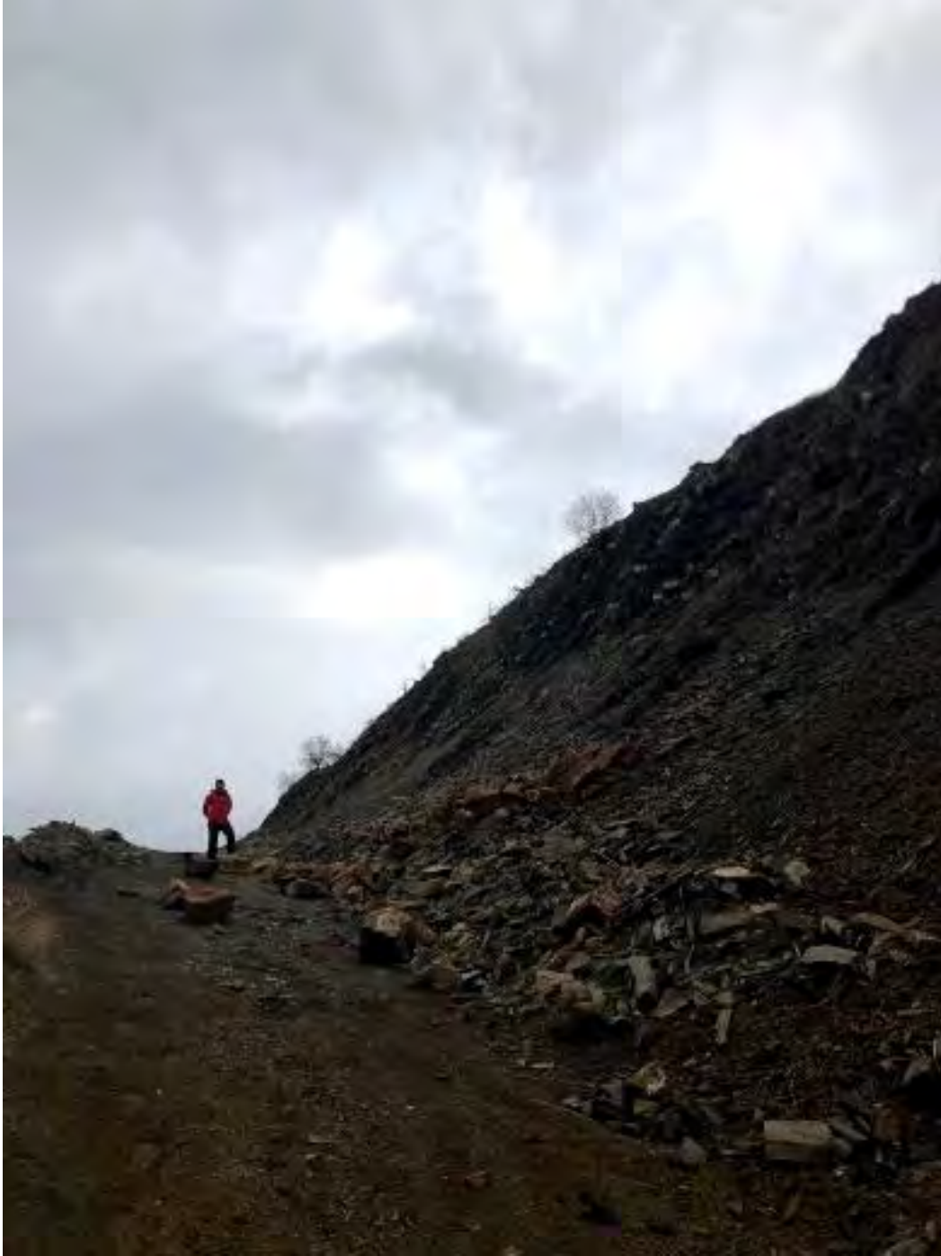
Figure 4.48. Rockfall at 13 th stop (upper bench) (38°31'41.5"N 39°27'60.0"E / 31.01.2020 / 16:10)
