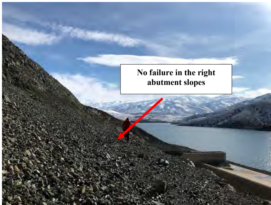
Figure 4.82. Right abutment natural slopes ( 38^{\circ}21'18.7''N 38^{\circ}36'36.0''E / 01.02.2020 / 10:25)
