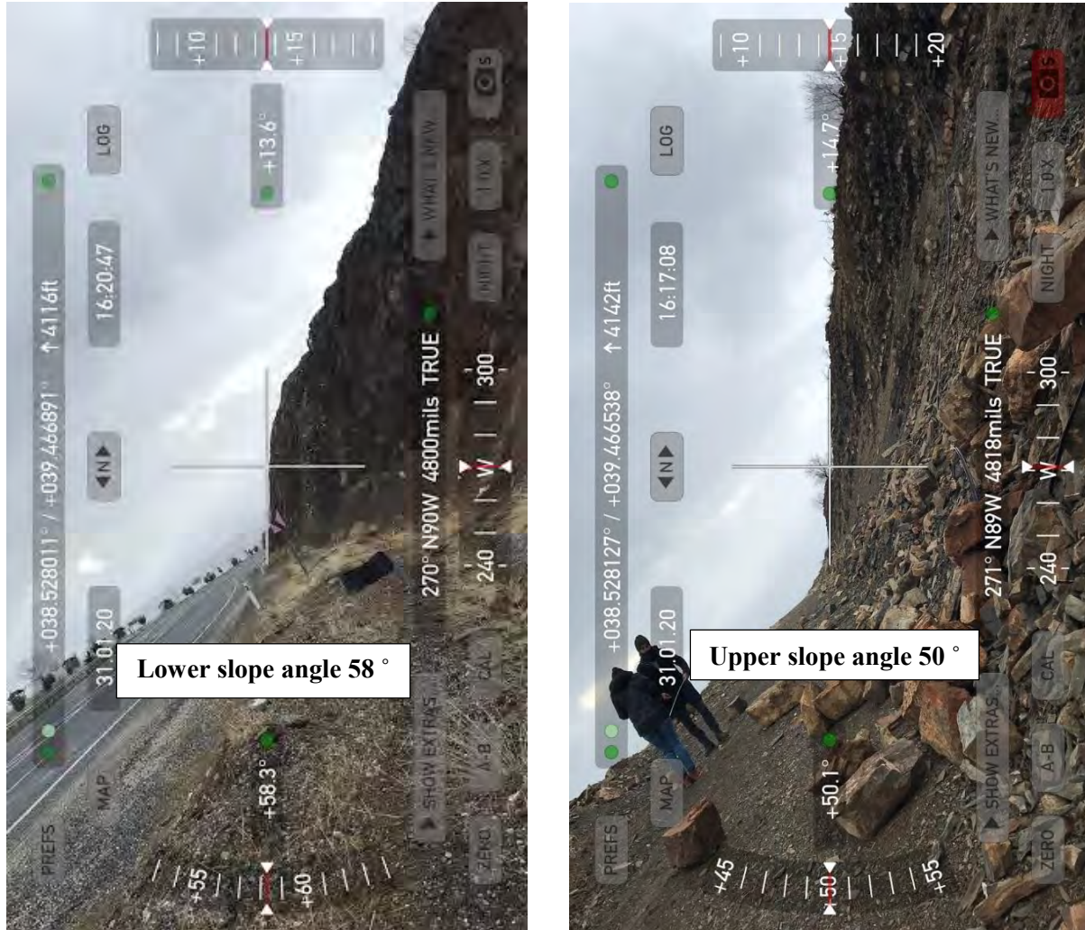
Figure 4.51. Rockfalls at 13 th stop (Slope angle determination) (38°31'40.8"N 39°28'00.8"E / 31.01.2020 / 16:20 & 38°31'41.3"N 39°27'59.5"E / 31.01.2020 / 16:17)
