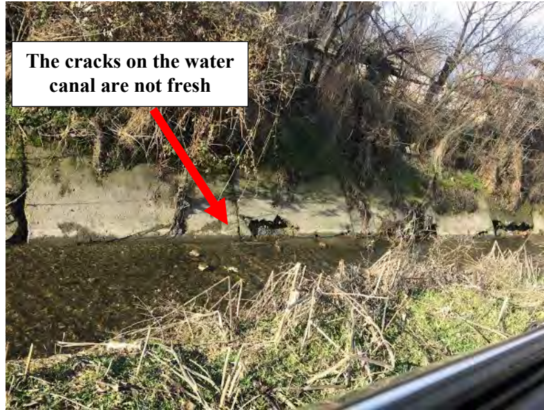
Figure 4.72. Water trench in Dolamantepe district of Battalgazi Village ( 38^{\circ}26'00.4''N 38^{\circ}21'44.1''E / 01.02.2020 / 9:25)
