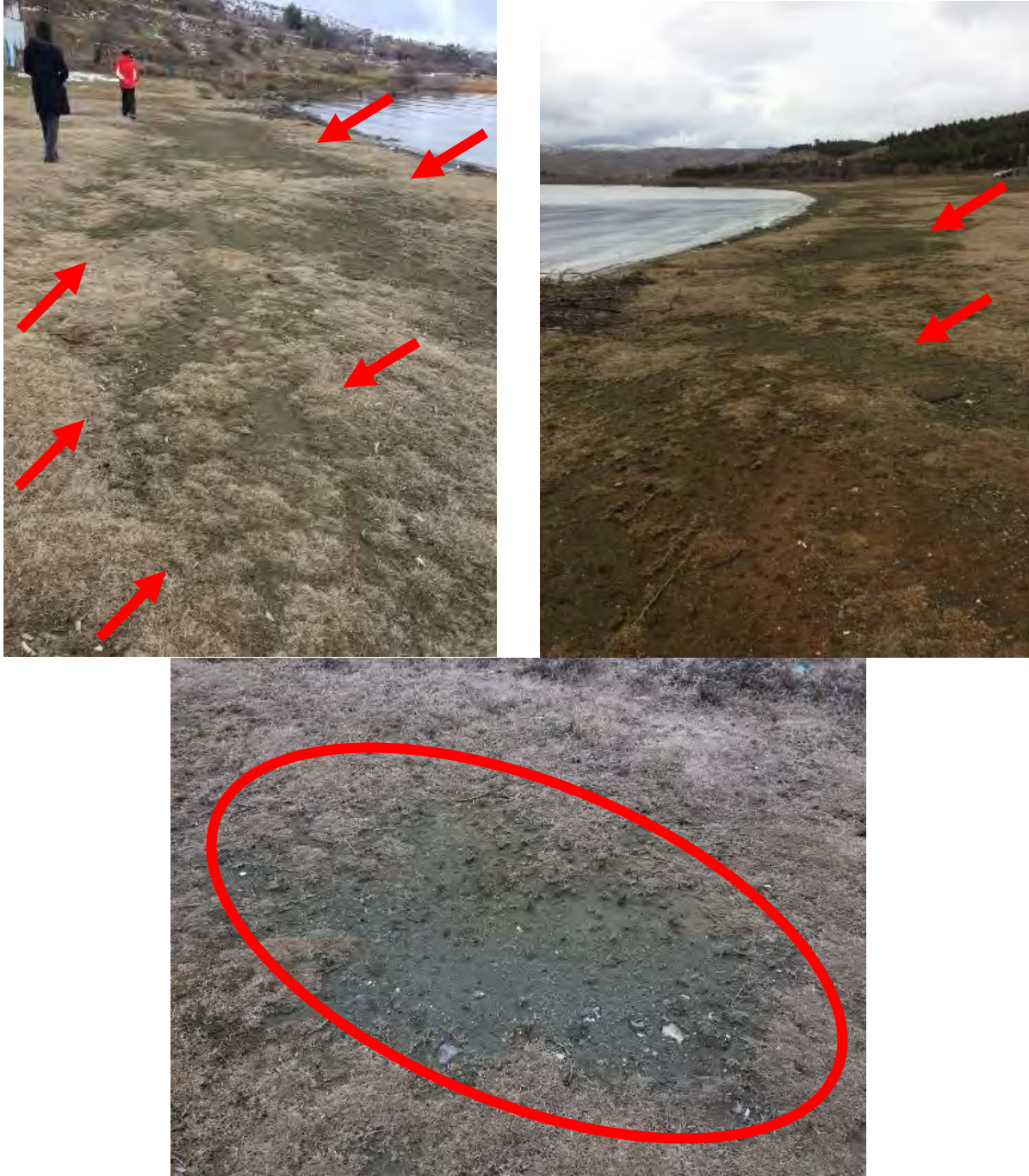
Figure 4.46. Sand boils observed
