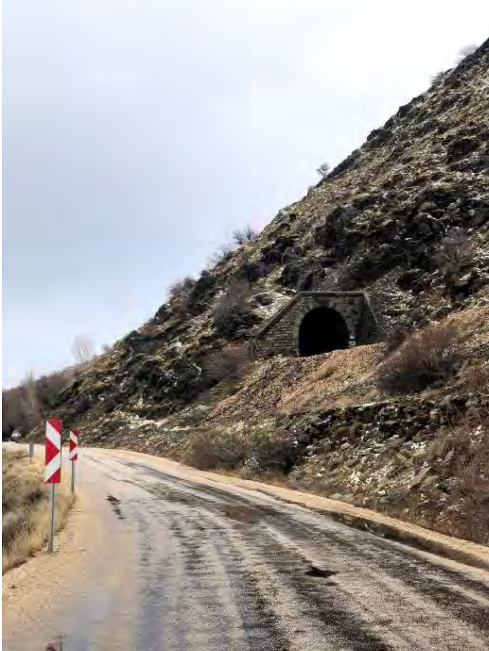
Figure 4.27. A view of the tunnel in Stop 5 (38°26'43.7"N 39°20'40.8"E / 31.01.2020 / 13:54)
