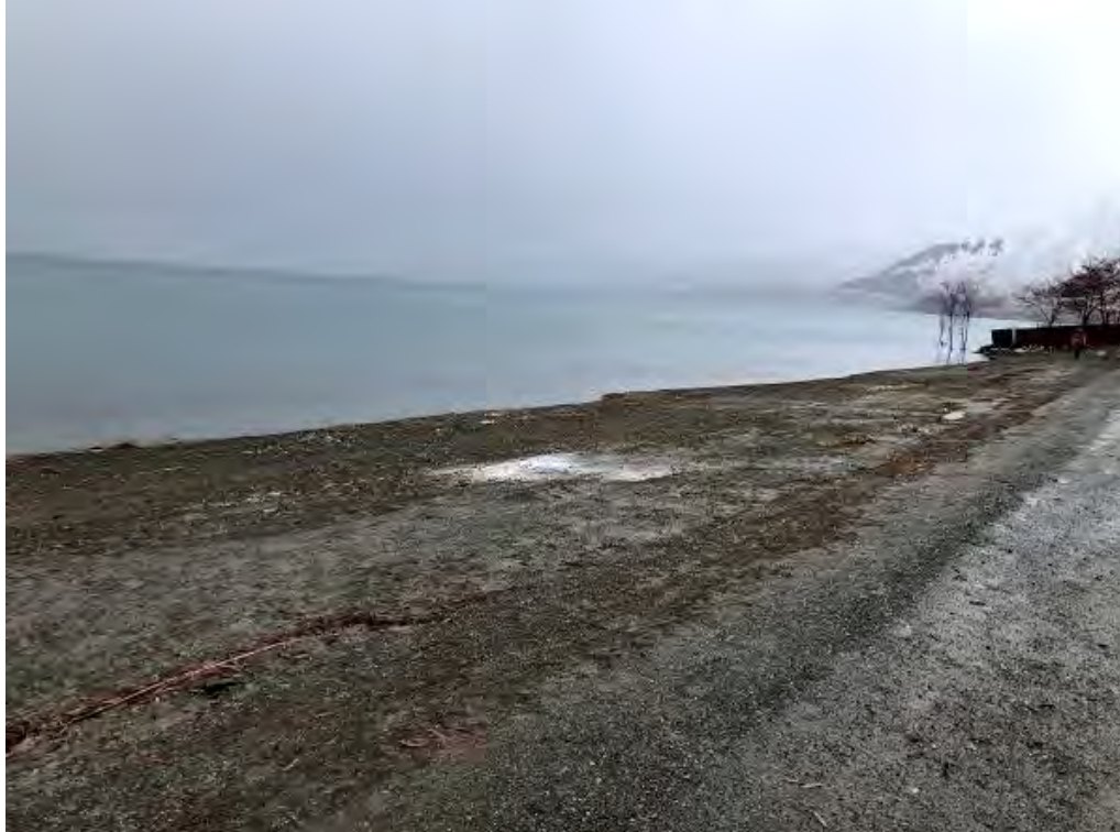
Figure 4.17. Seismically-induced lateral spreading on the beach of Hazar Lake ( 38^{\circ}26'48.4''N 39^{\circ}18'57.4''E / 31.01.2020 / 12:31 & 38^{\circ}26'50.1''N 39^{\circ}18'57.2''E / 31.01.2020 / 12:54)
