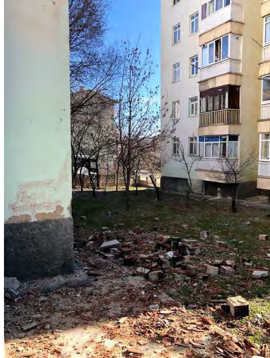
Figure 4.99. Cracks at the first floor, and fallen bricks ( 38^{\circ}39'31.9''N 39^{\circ}08'57.9''E / 01.02.2020 / 14:38 & 38^{\circ}39'32.0''N 39^{\circ}09'01.3''E / 01.02.2020 / 14:39)
