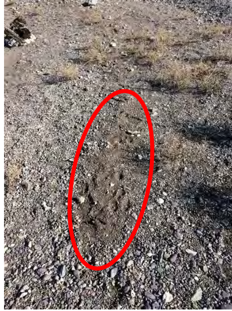
Figure 4.130. Surface manifestation of soil liquefaction at Kale Village shores (26 th stop) (38°25'20.2"N 38°45'33.2"E / 01.02.2020 / 12:25)
