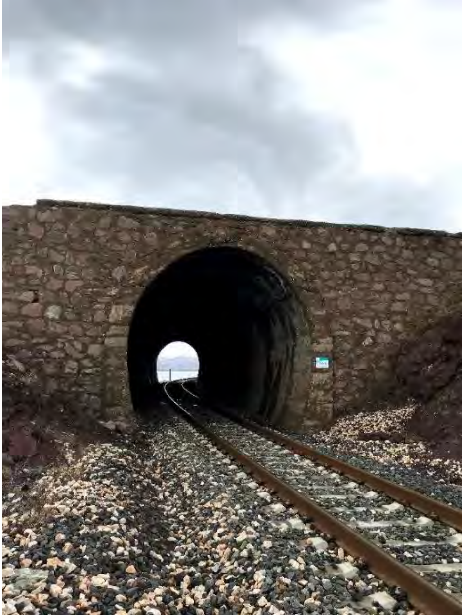
Figure 4.40. A railway tunnel and rails exhibiting no damage (38°28'52.8"N 39°27'18.2"E / 31.01.2020 / 15:08)
