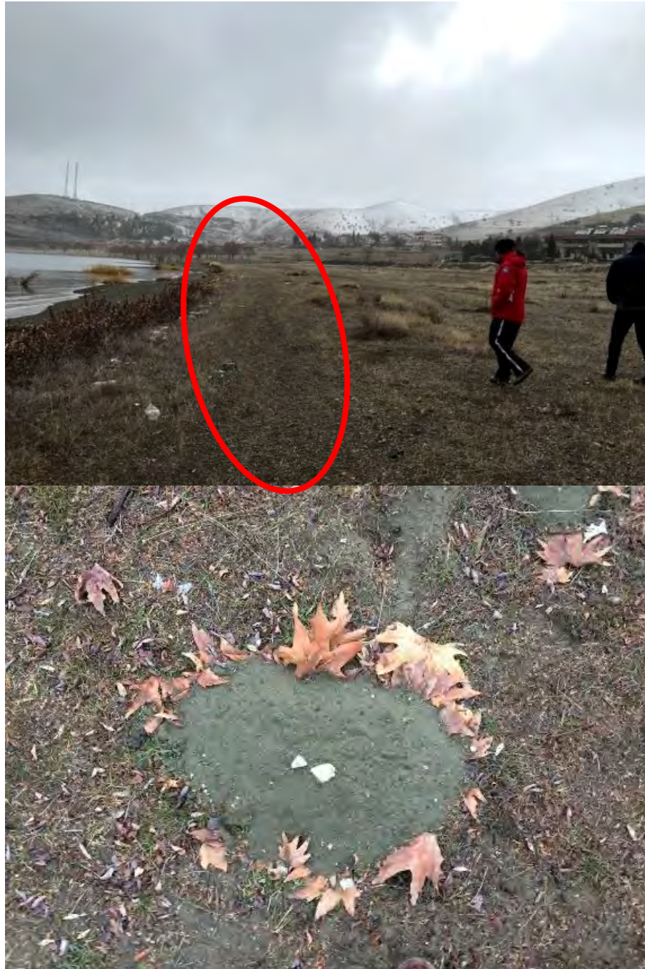
Figure 4.55: Seismic soil liquefaction-induced sand boils at Stop 15 (38°29'32.3"N 39°21'03.8"E / 31.01.2020 / 16:57 & 38°29'34.5"N 39°21'03.6"E / 31.01.2020 / 17:11)
