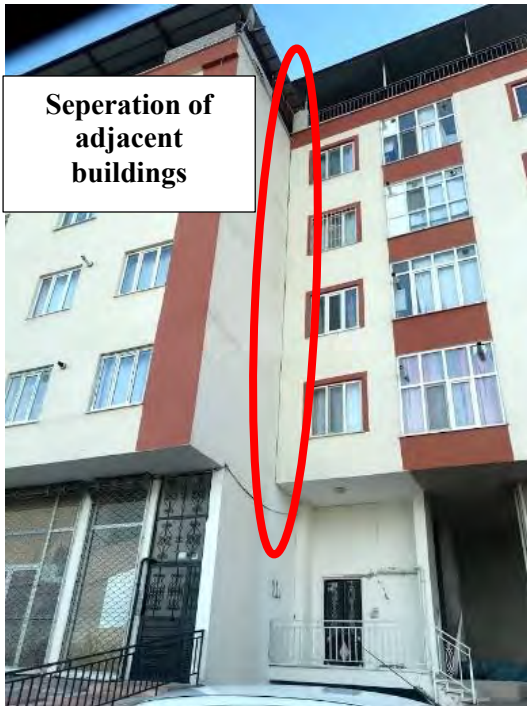
Figure 4.64. Separation of two adjacent buildings in Battalgazi Village ( 38^{\circ}25'40.4''N 38^{\circ}22'02.8''E / 01.02.2020 / 8:44 & 38^{\circ}25'35.4''N 38^{\circ}22'00.4''E / 01.02.2020 / 8:43)
