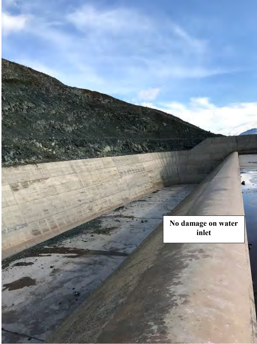
Figure 4.79. Spillway of Kapıkaya Dam ( 38^{\circ}21'17.2''N 38^{\circ}36'36.7''E / 01.02.2020 / 11:14)
