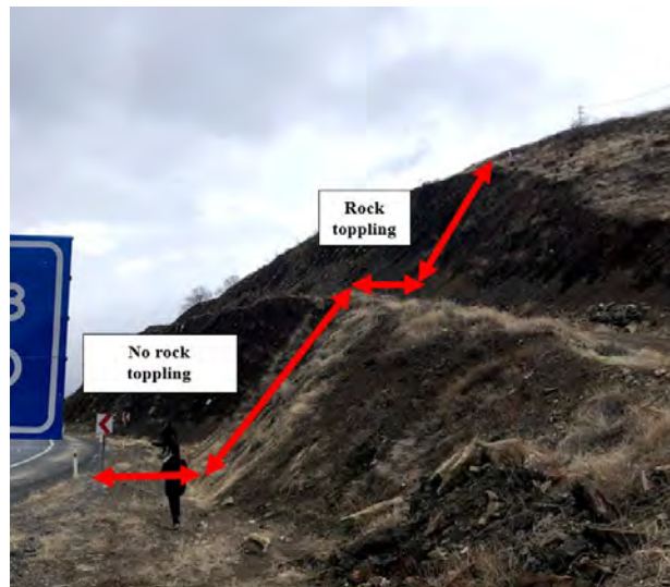
Figure 4.112. Cross section of the rockfall at 13 th stop ( 38^\circ31'40.3''N 39^\circ28'02.9''E / 31.01.2020 / 16:20)
