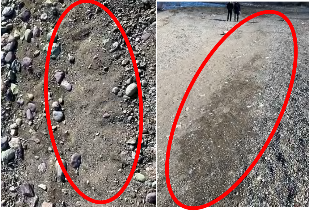
Figure 4.91. Seismic soil liquefaction-induced sand boils at Kale shore ( 38^{\circ}25'15.2''N 38^{\circ}45'32.2''E / 01.02.2020 / 12:32 & 38^{\circ}25'15.2''N 38^{\circ}45'23.9''E / 01.02.2020 / 12:45)
