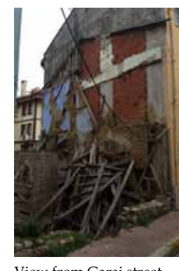
View from Garaj street
