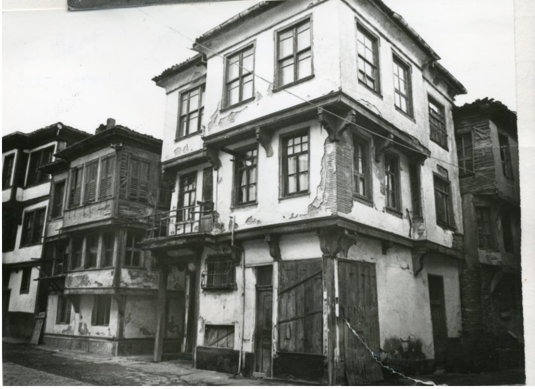
Figure 2.67. House on İskele Street Lot no: 2206/3 (Photo taken from Bursa KVKBKM archive)
