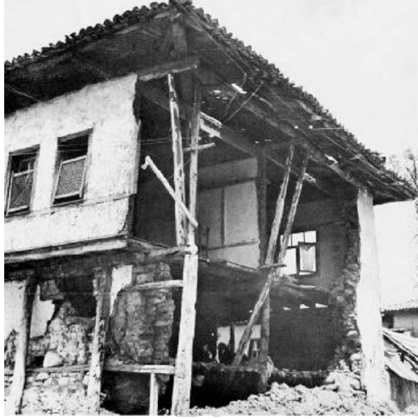
Figure 4.2. Traditional house in Örencik, after 1970 Gediz earthquake, destruction of a two-story-high stone masonry wall of a house while the rest of the timber frame section of the structure still stands (Şahin Güçhan, 2007, p.844, fig no:3)
