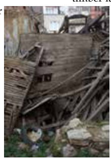
Floor girders and floor boards
