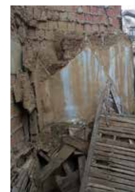
Timber frame wall with mudbrick infill and mudplaster
