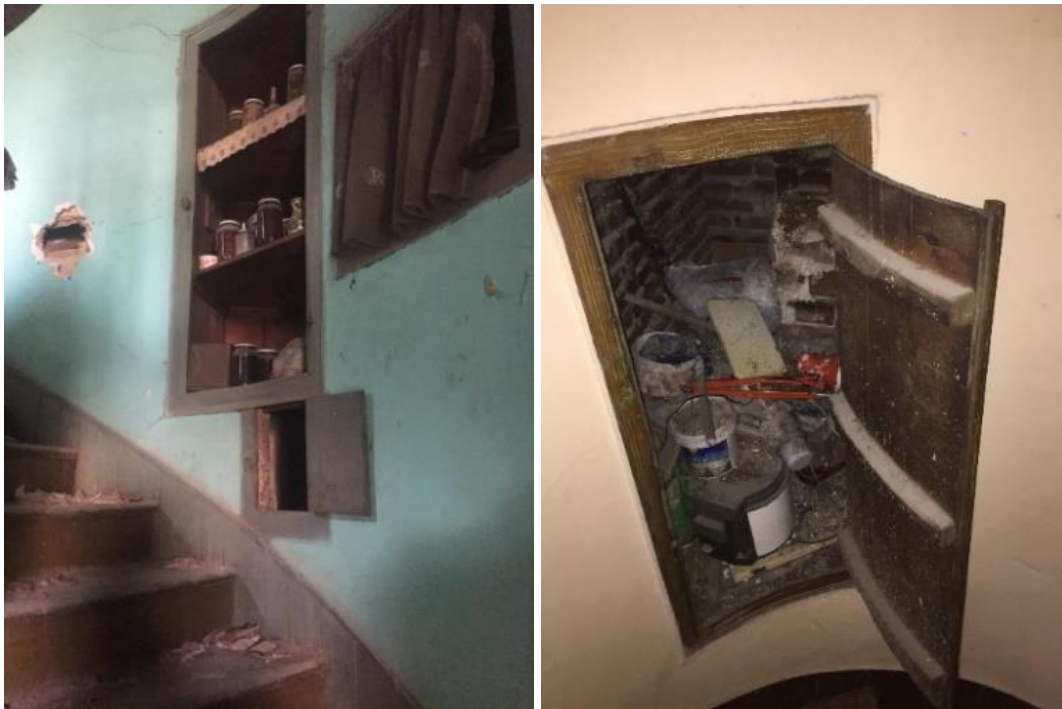
Figure 2.80. Niches on the curvilinear timber frame walls of the staircases
