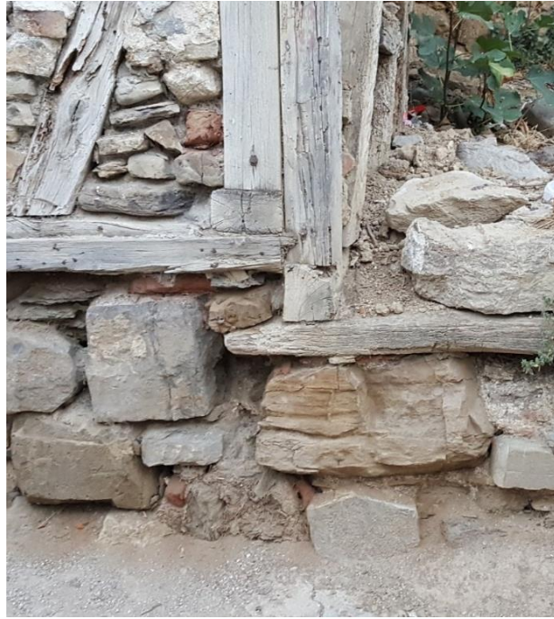
Figure 3.28. Unique masonry – timber frame connection detail of two attached buildings.
