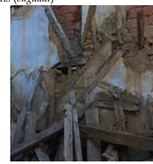
Traces of the staircase
