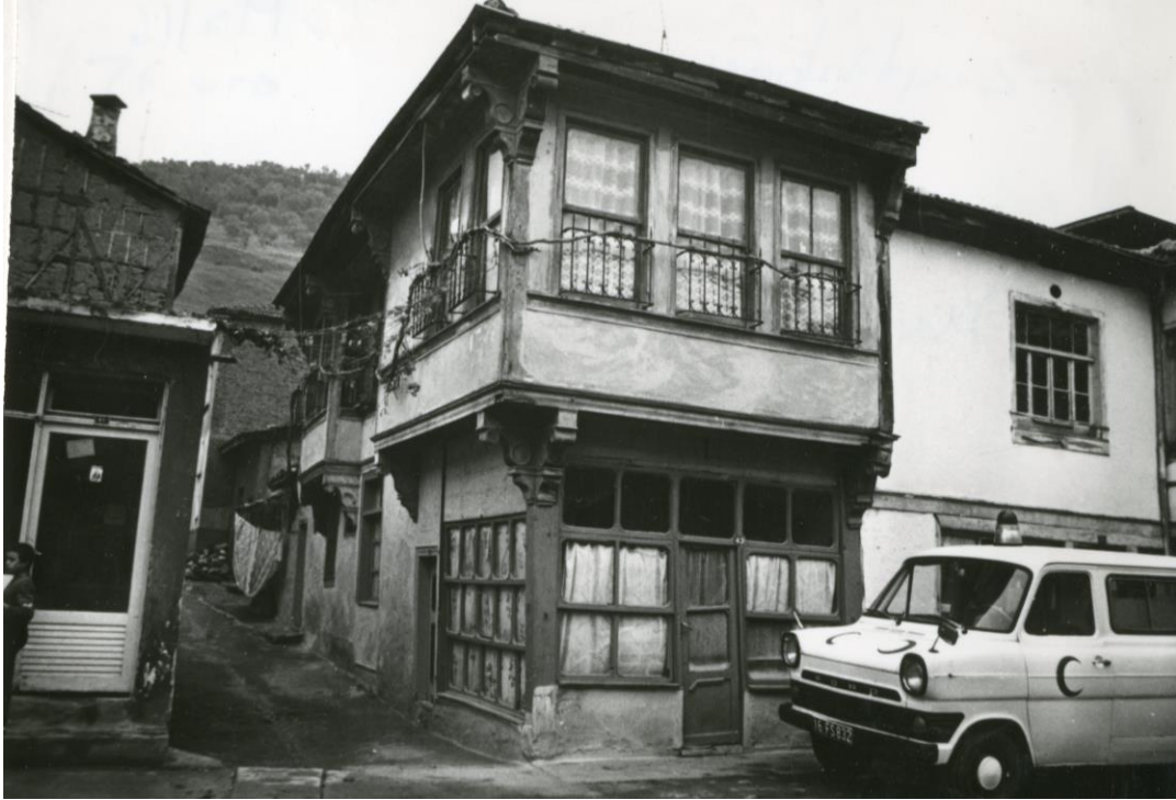
Figure 2.66. The house before restoration, İskele Street, Tirilye Lot no: 2226/3.
