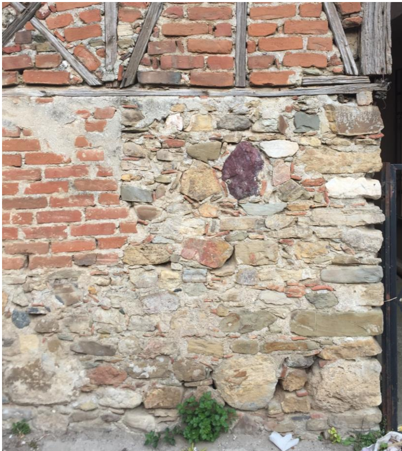
Figure 3.6. Rubble stone masonry wall coursing example (Lot no: 2167/1)
