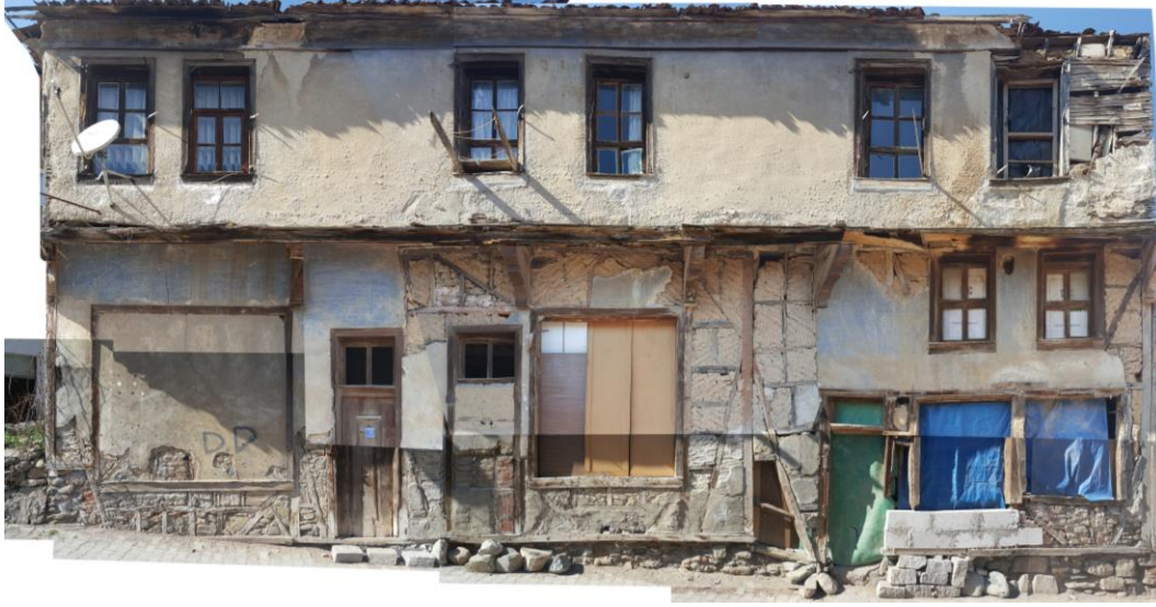
Figure 2.60. Façade of House No:5 (Cami St, Lot no:2186/)
