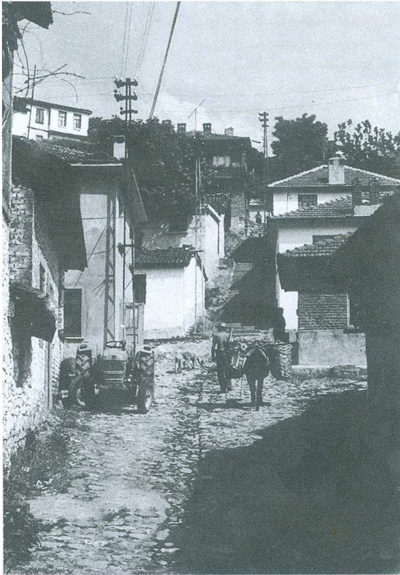
Figure 2.17. The authentic street pavement of Tirilye street, which is lost today.
