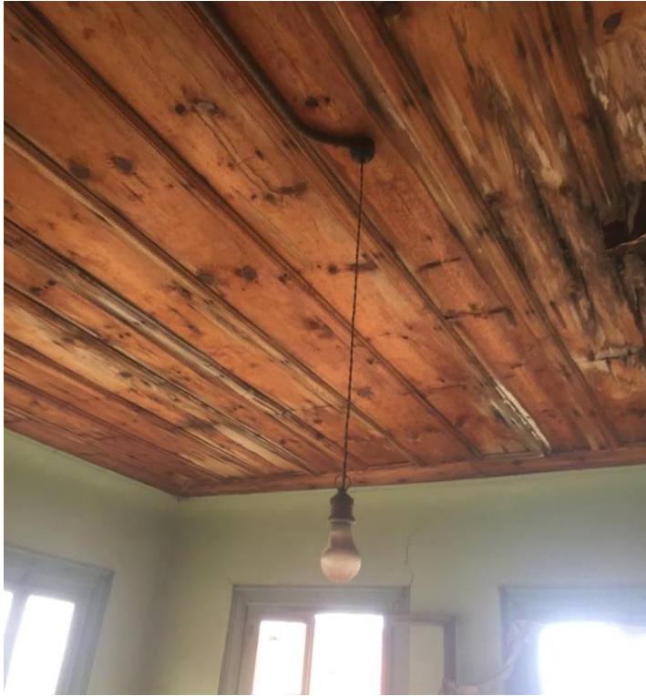
Figure 2.77: Common type of timber ceiling, House No:1
