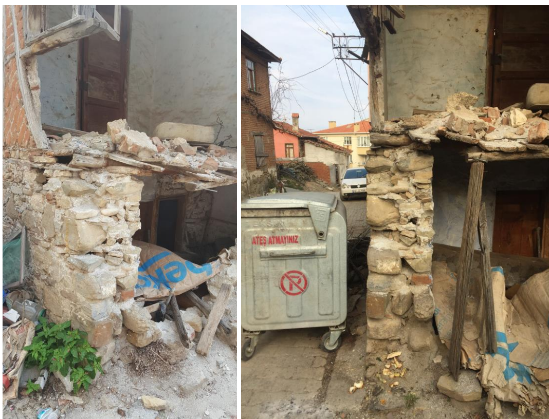
Figure 3.12. Masonry wall coursing without lintel (Lot no: 2167/1)
