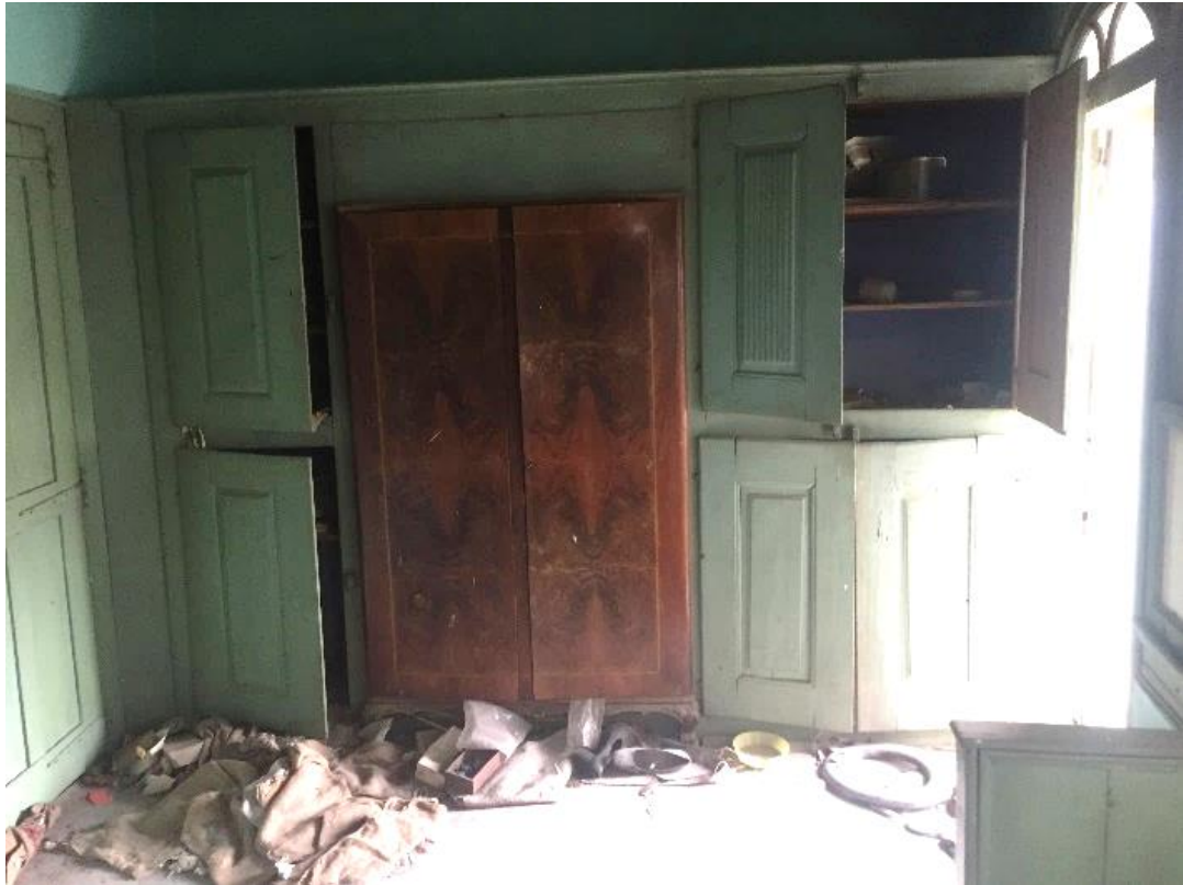
Figure 2.81. Cupboard covering the sidewall of the room on the first floor
