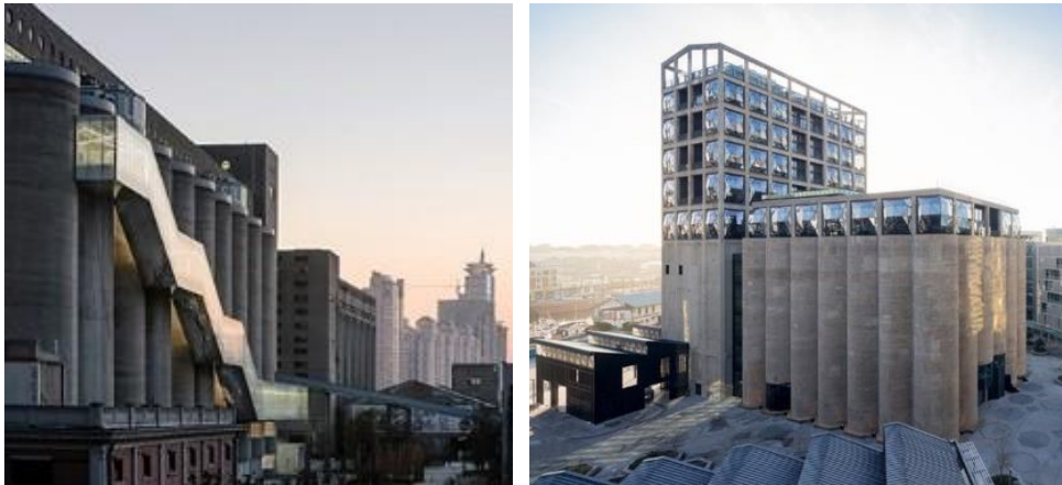
Figure 2.23. Examples of the preserved-bins designs matching with the corresponding illustrations above. From left to right: Minsheng Wharf by Atelier Deshaus, Zeitz Museum of Contemporary Art in Cape Town by Heatherwick Studio.
