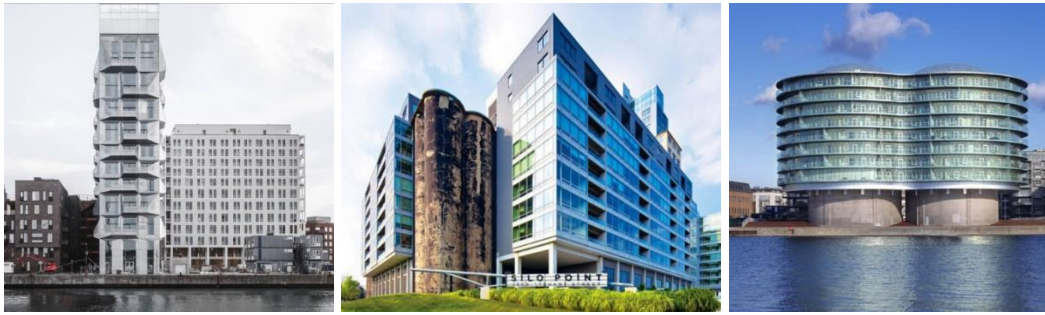
Figure 2.19. Examples of the additions-on-bins designs, matching with the corresponding illustrations above. From left to right: Housing in Denmark by Cobe, Residence in Baltimore by Parameter Inc, Housing in Denmark by MVRDV.
