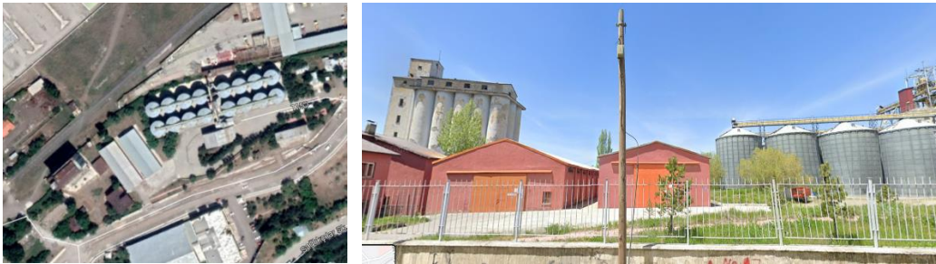
Figure 3.11. The old abandoned reinforced concrete silo and the relatively newer steel silo are on the same campus in Erzurum.
