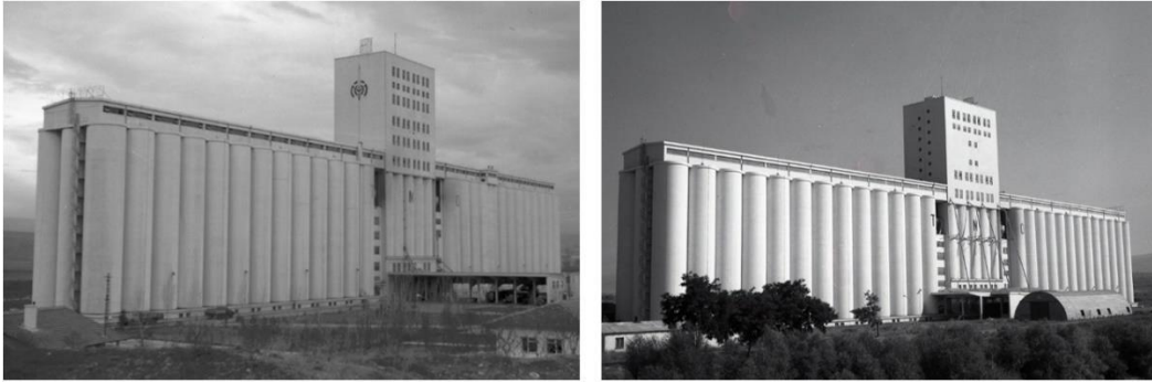
Figure 3.14. Ankara Güvercinlik Silos photographs from the north (left) and south (right). Establishment in 1958 by the English company of Simon Handling Engineers Ltd.
