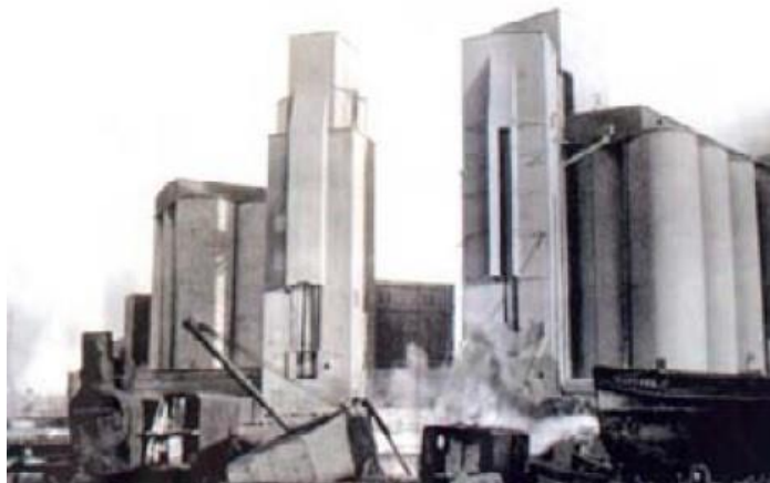
Figure 2.9. American Elevator, first concrete elevator in Buffalo (1906).
