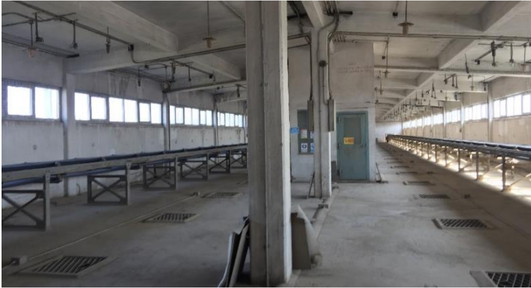
Figure 4.22. Portable equipment in conveyor floors, with wheels (top left) or glides through the belts (top right) and the spacious upper conveyor floor with only belts and pipes (bottom) (Author, 2020).
