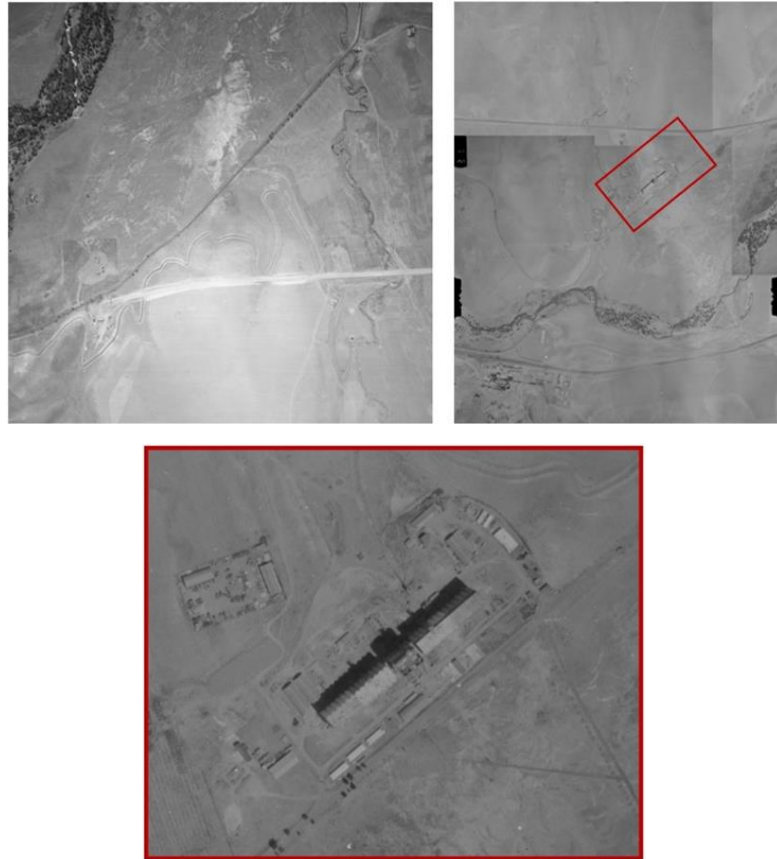
Figure 3.23. Before and after the construction of the silo, the first photograph is from 1952, and the second and third photographs are from 1957.
