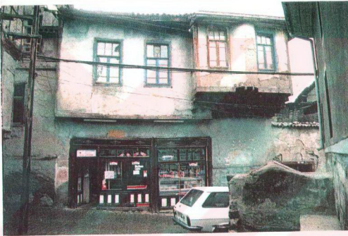
2) Kalekapısı St., 10, Kaleiçi, new window opening in ground floor for new function
