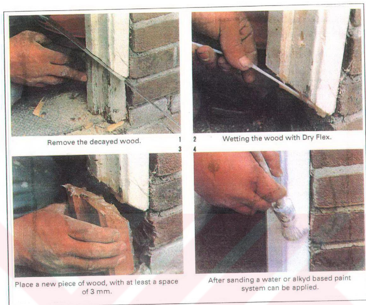
Figure 5.14. Insertion of a New Timber to Renew a Decayed Section (Window Care System™)
