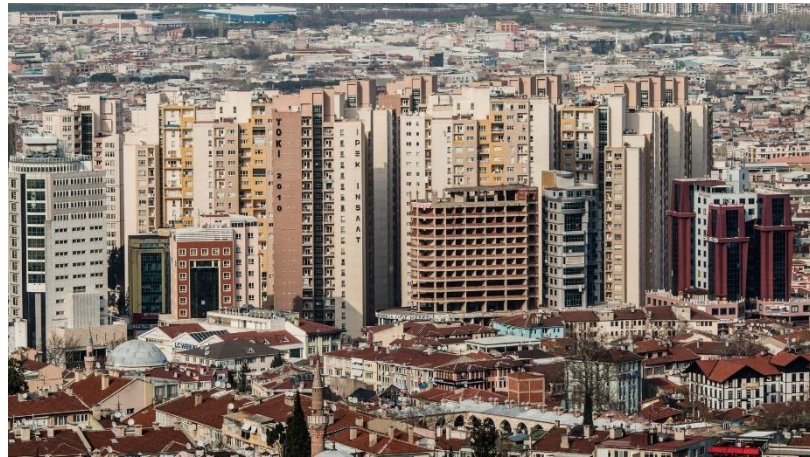
Figure 14. The general view of Doğanbey neighborhood and TOKİ dwellings
