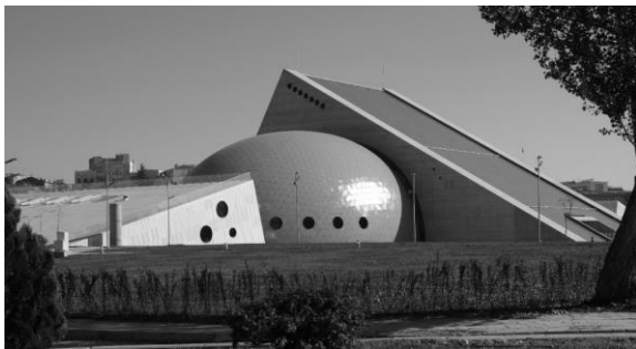
Figure 52. CSO Concert Hall (New) By Uygur Architects. 2021. 287
