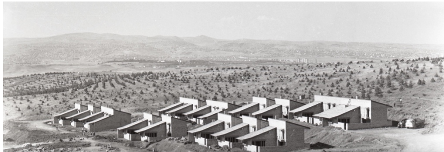
Figure 2.10. Construction site photograph of the METU lodgings 63
