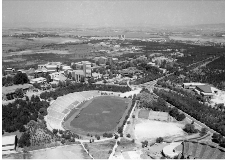
Figure 3.2. Aerial view of the METU campus 93
