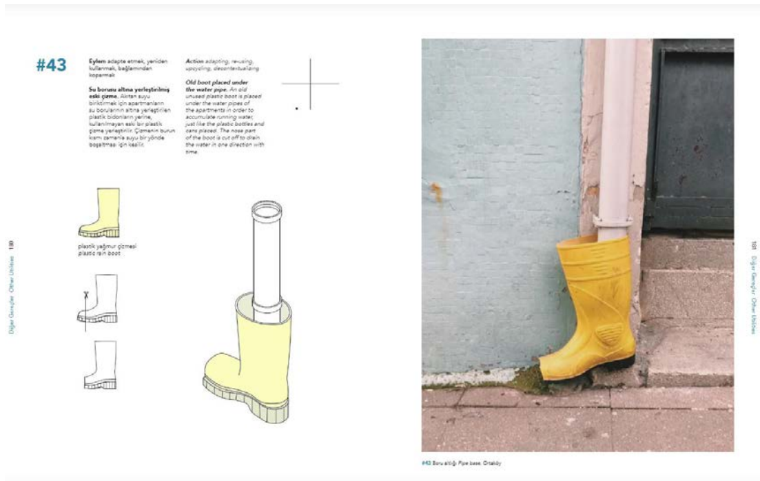
Figure 2.6: A discarded plastic boot is used to redirect the flow of water. (Horsanalı, 2018)
