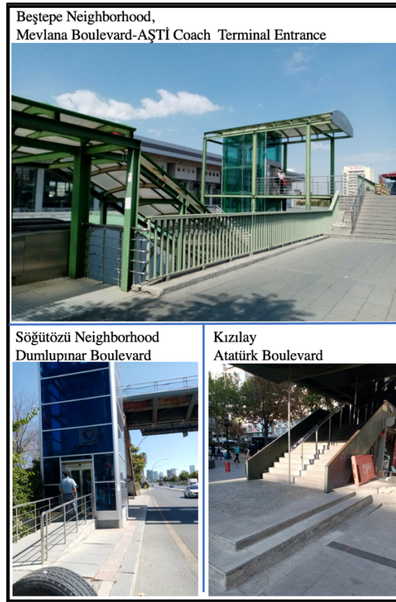
Figure 5.42. Example Views from Overpass and Underpass (Photographs Taken During Fieldwork)
