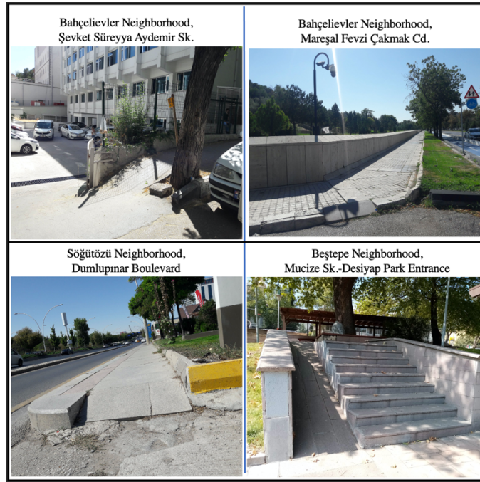
Figure 5.32. Example Images of Problematic Ramps in terms of Slope (Photographs Taken During Fieldwork)
