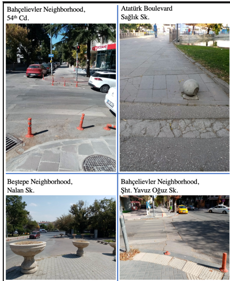
Figure 5.39. Permanent Barriers to Access Crossing: Fixed Bollards and Street Furniture to Prevent Motorized Vehicle Access (Photographs Taken During Fieldwork)
