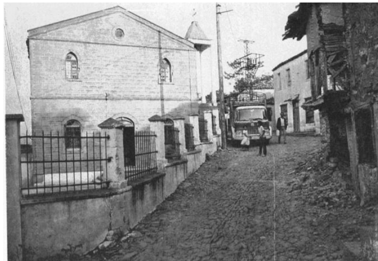
Figure 3.24. Dereköy, the Church of Panagia in 2020 (above); an old photograph of the Panagia Church (below) (Chalkia 1992, p. 322)
