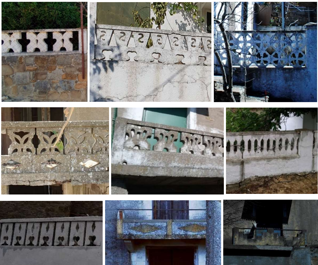
Figure 3.58. Dereköy, different types of balustrades in courtyards and balconies
