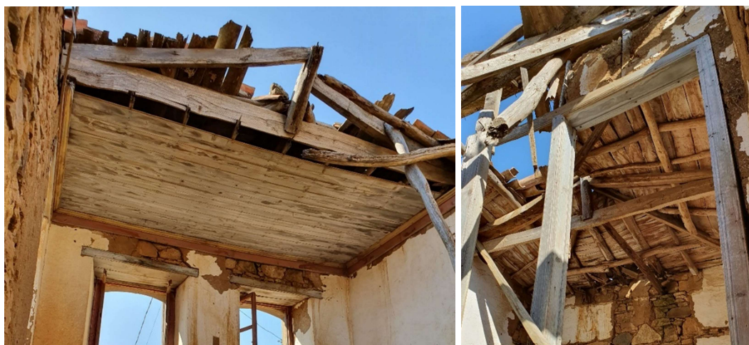
Figure 3.53. Dereköy, structural system of a gabled roof
