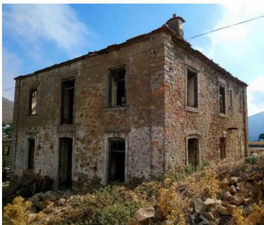
Figure 3.62. Dereköy the former karakoli building
