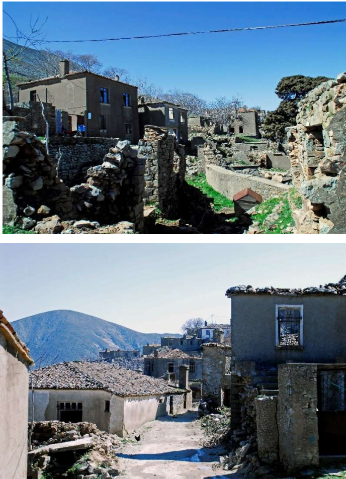
Figure 3.38. Derelict houses in Dereköy
