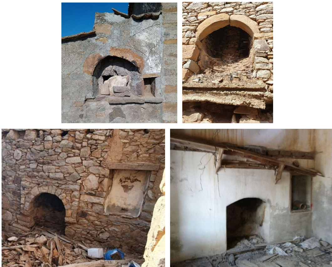
Figure 3.59. Dereköy, fireplaces in different courtyards (above); a fireplace and a niche on the ground floor (below left); a fireplace on the upper story (below right)
