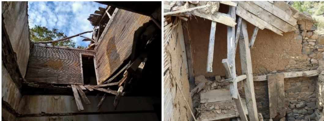
Figure 3.50. Dereköy, bağdadı partition walls on the upper floor (left); the plastered wall of the upper floor (right)
