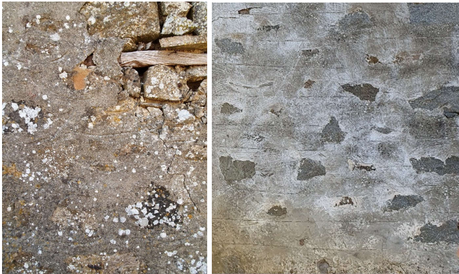
Figure 3.48. Dereköy, patterns of plaster applications on the exterior.
