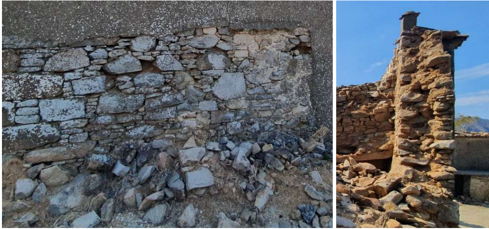
Figure 3.47. Dereköy, Traditional masonry walls
