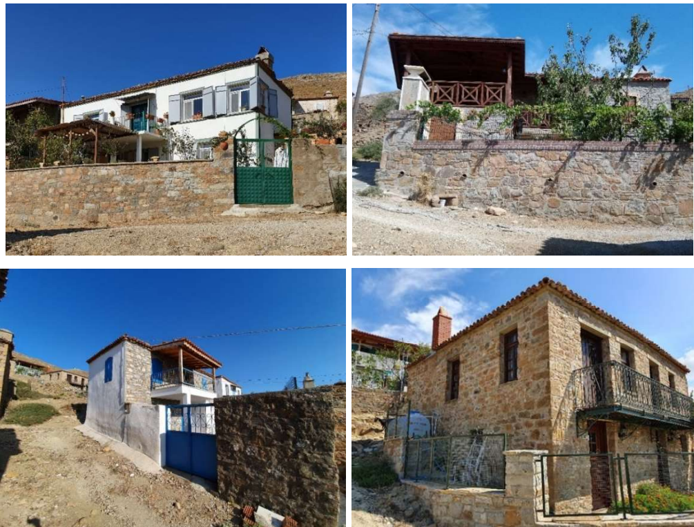
Figure 3.66. Dereköy, examples of renovated houses
