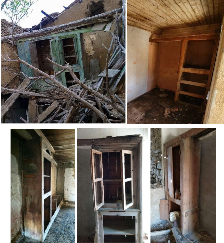
Figure 3.60. Dereköy, timber closets on the upper floor
