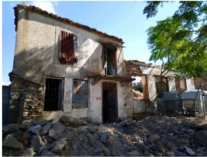
Figure 4.3. Derelict buildings in Dereköy
