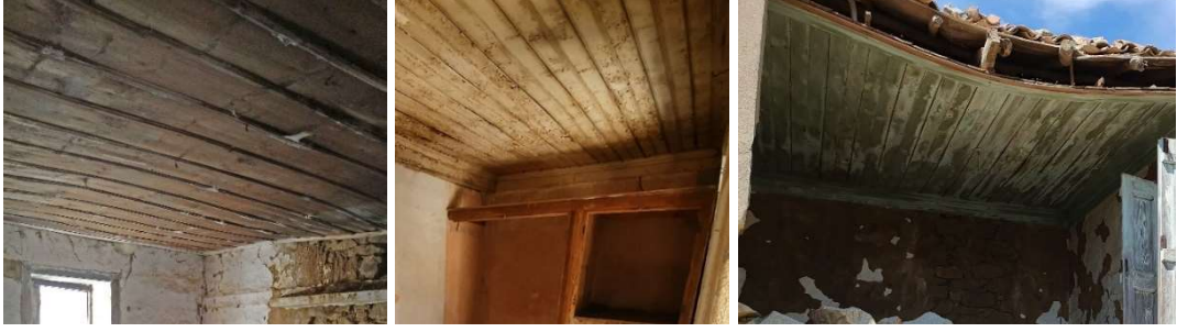
Figure 3.54. Dereköy, timber ceilings
