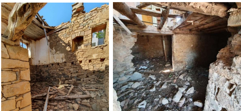
Figure 3.51. Dereköy, putlog holes (left); timber floor beams (right)
