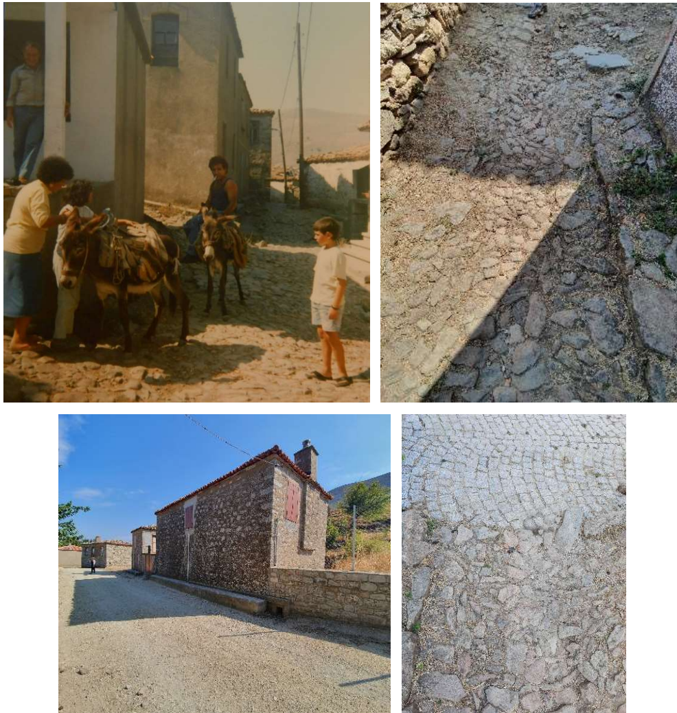
Figure 3.18. An old photograph showing the authentic kalderimi pathway (above left) (URL 48); a preserved kalderimi in 2020 (above right); a dirt street (below left), kalderimi and a new stone pavement (below right)
