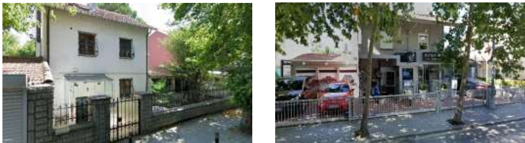
Figure 5.19. Examples of Residential and Commercial Buildings on Lale Street
