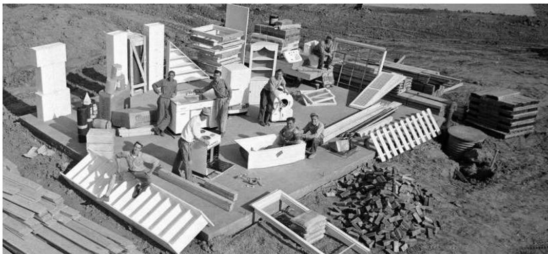
Figure 4.10. Levittown House Components – Building Site
