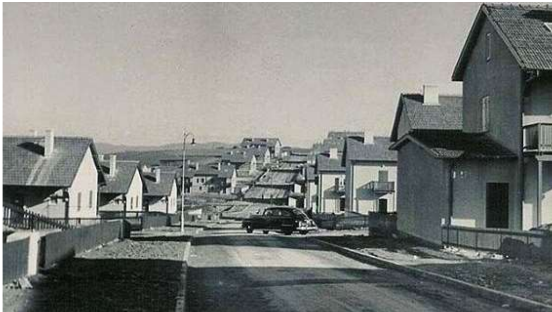
Figure 5.17. Levent Street View Shows the Silhouette Created by the Plot-Block System
