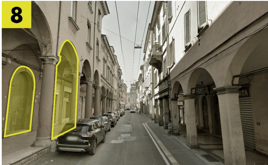
Figure 4.25: Application of echoes on arches of the vaults and gates (Google Earth, n.d.)
