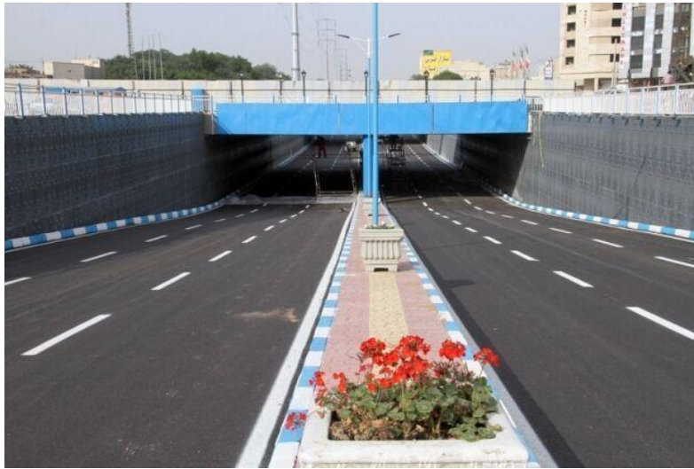
FIGURE 3. the underpass bridge in Tehran.
