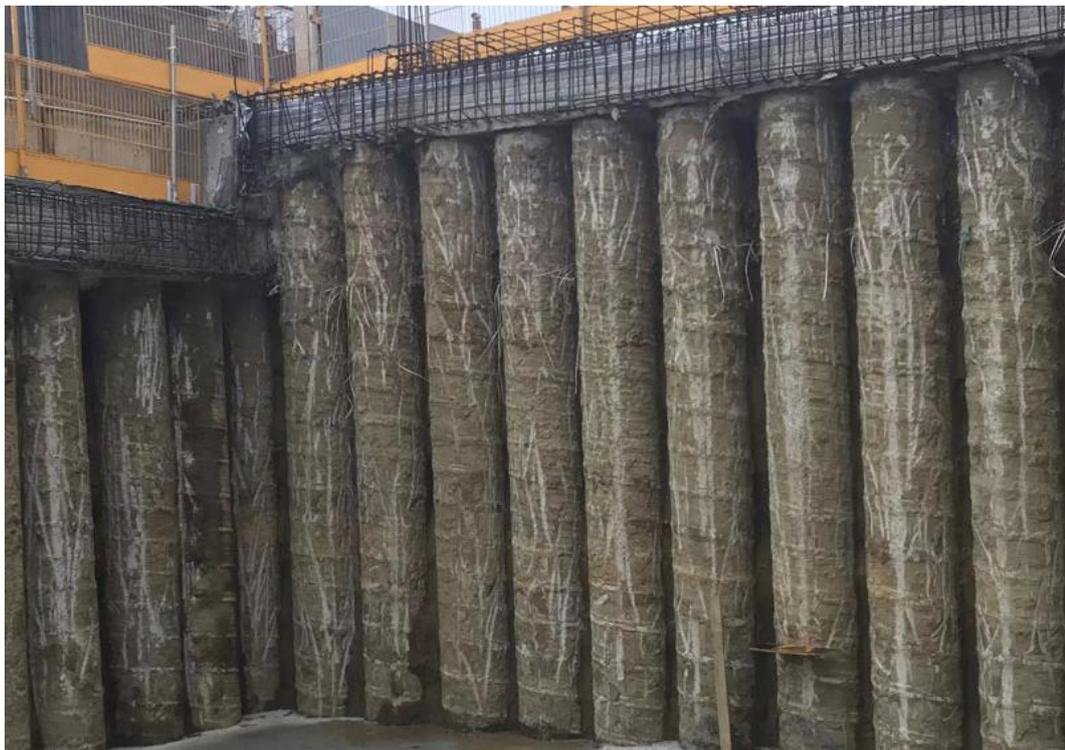
Figure 2.2. Cantilever Bored Pile Excavation System
