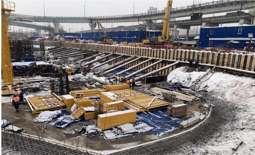
Figure 2.14. Excavation Supported with Rakers
