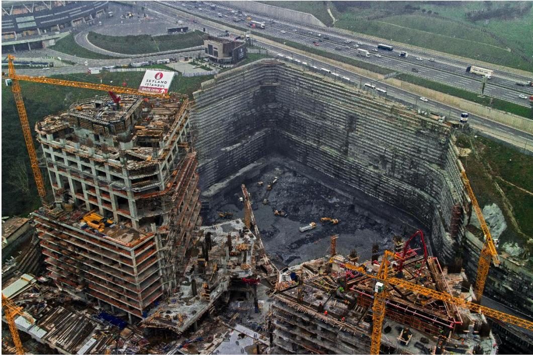
Figure 2.6. Multi-layered Anchored Wall System
