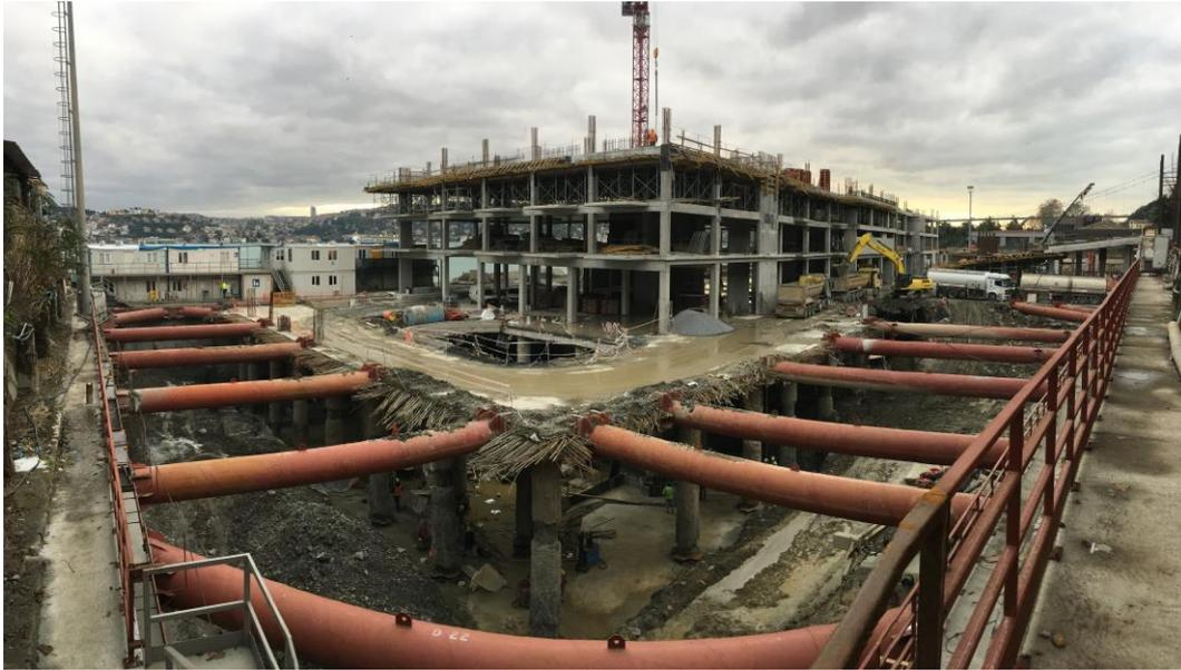
Figure 2.15. Top-Down Excavation System
