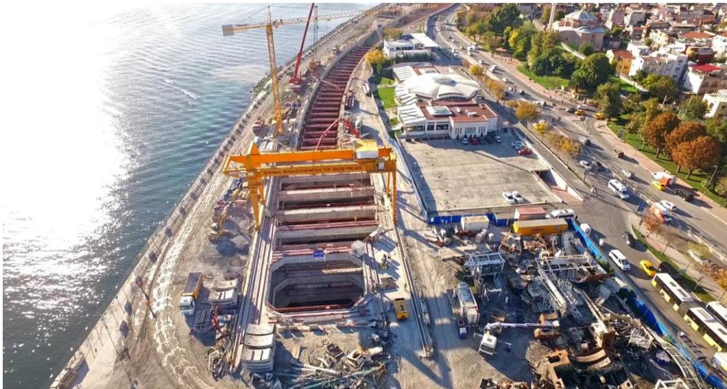
Figure 2.13. Excavation Supported with Struts
