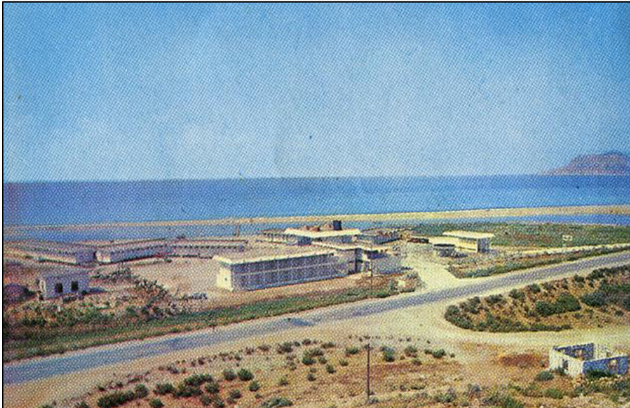
Figure 28. General view of Alantur Motel, D400 Motorway and the Mediterranean Sea (Personal archive of Feyzi Açıklın)
