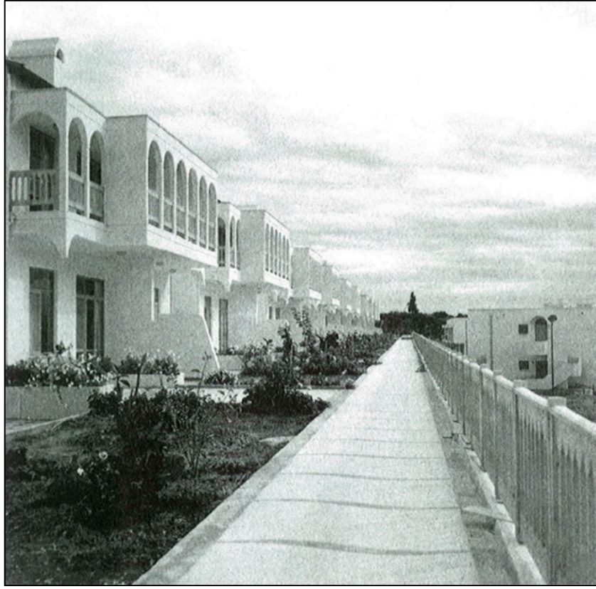
Figure 47: Fuğla 1 Holiday Houses Complex, 1981-1982 (Aydan Erim, “Bir Mimar: Nejat Ersin”, Mimarlık , no. 257(1994).)
