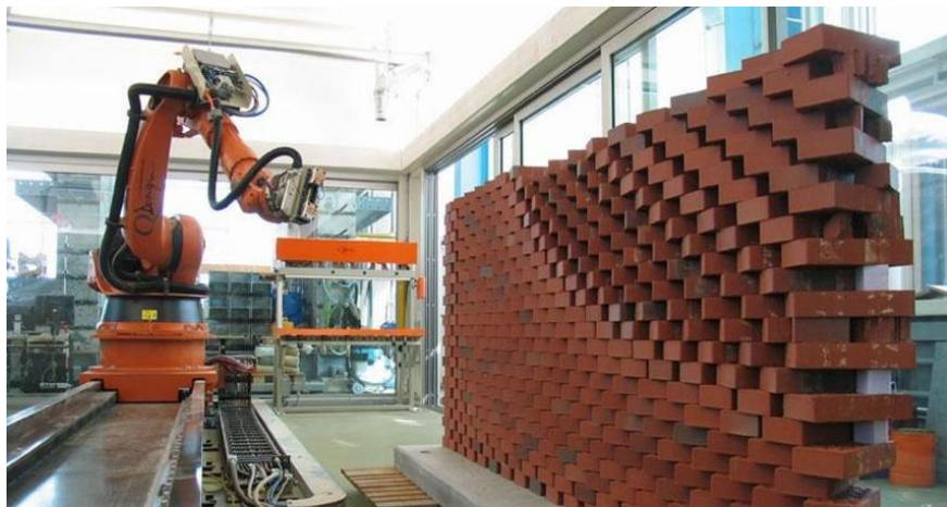
Figure 3: A robotically constructed brick wall. (Gandia, 2018)
