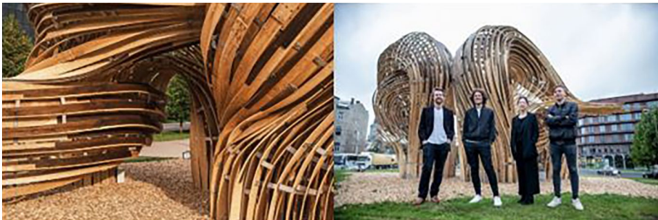
Figure: 10 Technological interventions interact with natural material reality- Steam-bent hardwood using primitive hand tools augmented with the precision of intelligent holographic guides/Steampunk Tallinn Architecture Biennale 2019 – Beauty Matters (Source: https://www.archdaily.com/926191/steampunk-pavilion-gwyllm-jahn-and-cameron-newnham-plus-soomeen-hahm-design-plus-igor-pantic ).
