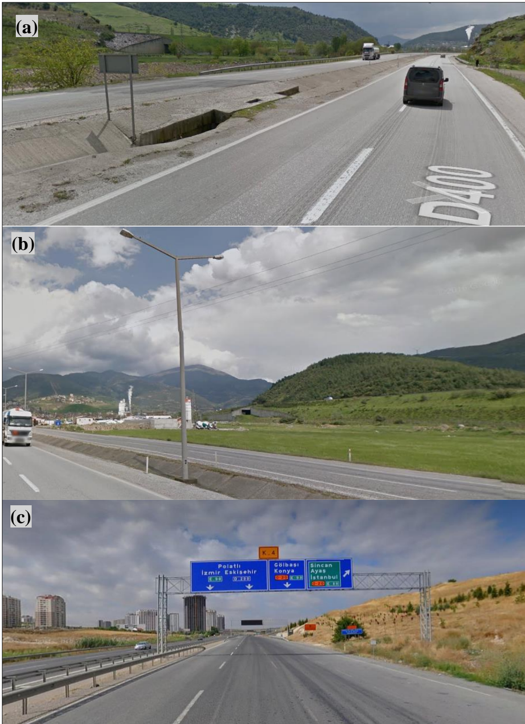
Figure 7.1 (a) Drainage ditch (b) Lighting pole (c) Signal gantries in the median of state roads
