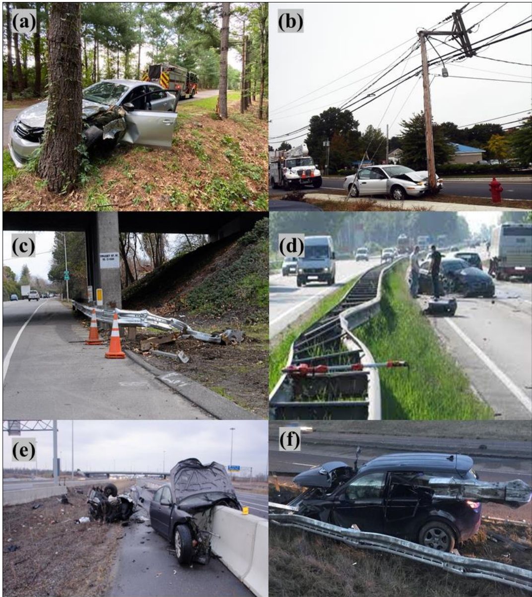
Figure 1.1 (a) Crashing into a tree (b) Crash to utility pole (c) Prevent reaching bridge pier (d) Prevent crossing median (e) Faulty terminal design of concrete barrier (f) Faulty terminal design of steel barrier
