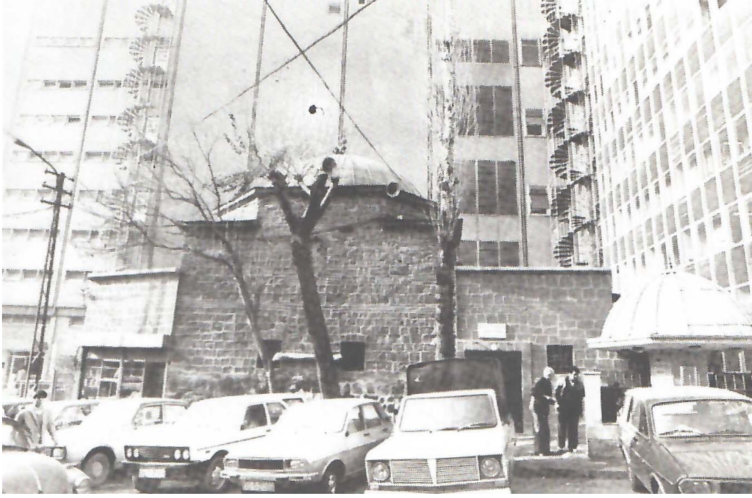
Figure 70. Hallaç Mahmud Masjid, No Date (Source: Şahin, 1992)
