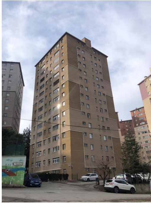
Figure 3.1. The selected building called 14 th block building in Ankara, Turkey.
