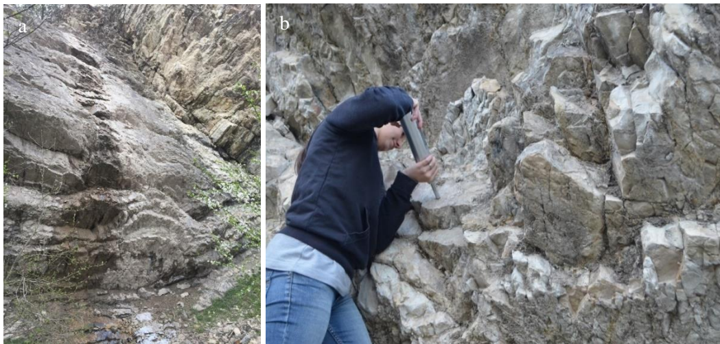
Figure 18: a) The surface drainage flow observed in the spring season, b) Schmidt hammer measurement in the field
