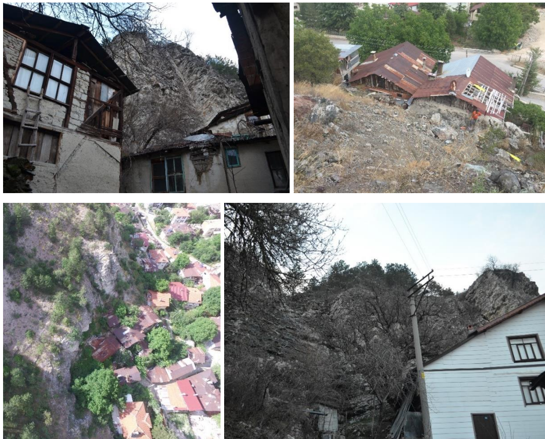
Figure 5: Views from the rock mass of the western side of the Mudurnu valley and houses under threat
