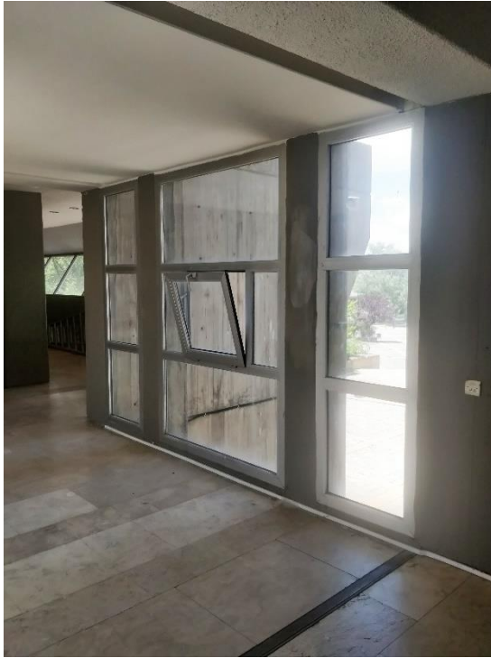
Figure 3.5: Interior of bridge with bottom hung casement window
