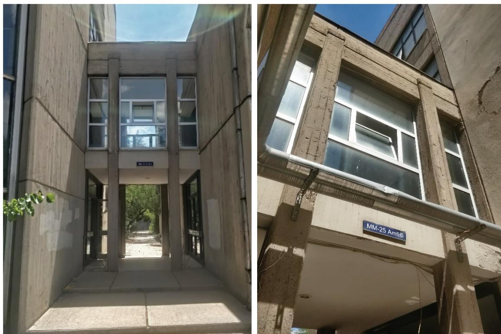
Figure 3.4: Bridge from MM Building to amphitheater section
