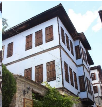
Buildings in Average Condition
