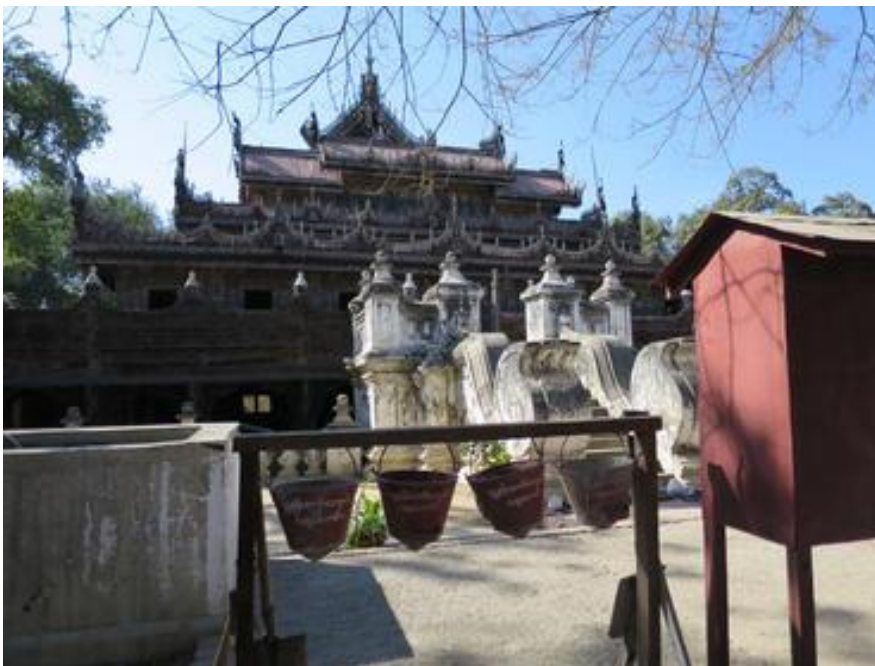
Fire suppression shovels and sand buckets at Shwe-nandaw Kyaung in Mandalay, Myanmar ( https://www.wmf.org/fire )
