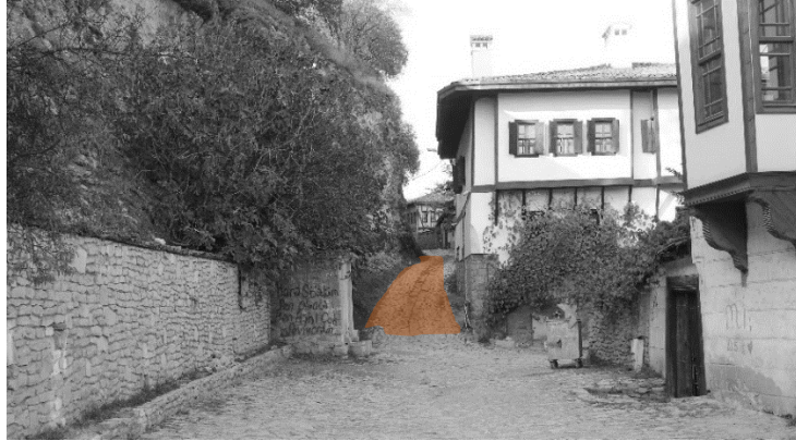
Figure 72 Gümüş Street and Hükümet Street Junction, the width is less than 4 meters, and the slope is more than 15 %. (Uluç, 2020)
