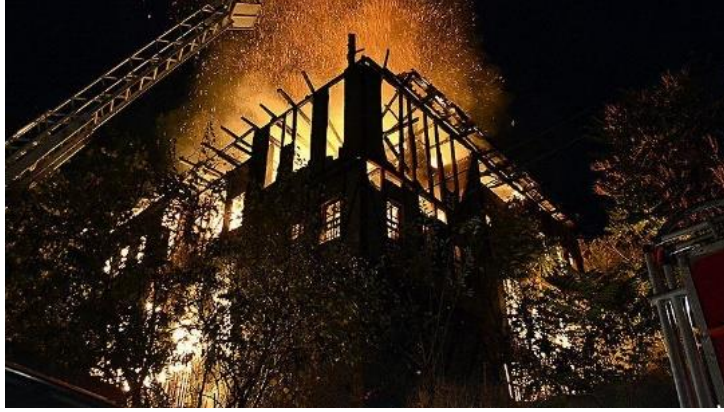
Figure 69 Historic Building Fire on 26 September 2016 [URL 45]
