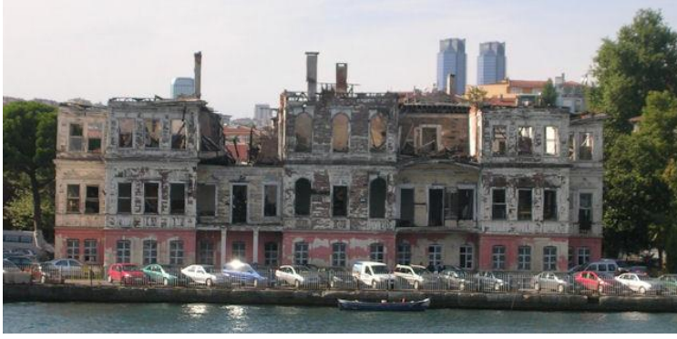
Figure 5 Gazi Osman Paşa Primary School Fire on 13 July 2002 (Atılgan, 2013)
