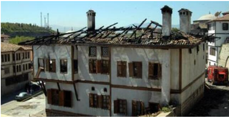
Figure 76 Historic Building Fire on 3 May 2010 [URL 43]
