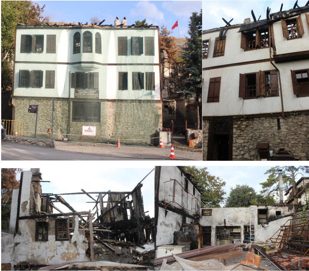
Figure 55 After Fire at Kadıoğlu Konak and the traditional building next to it on 23 July 2020 (Uluç, 2020)
