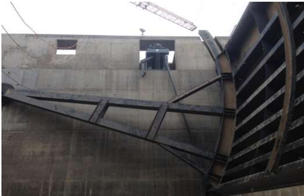
Figure 3.9: Radial Gates and Its Lifting Mechanism ( www.vortexhydradams.com )
