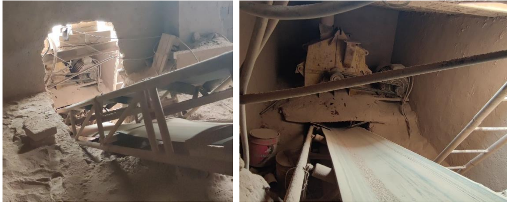
Figure 4.4. Second mill system to grind and crush the rubble into smaller pieces for the refractory brick
