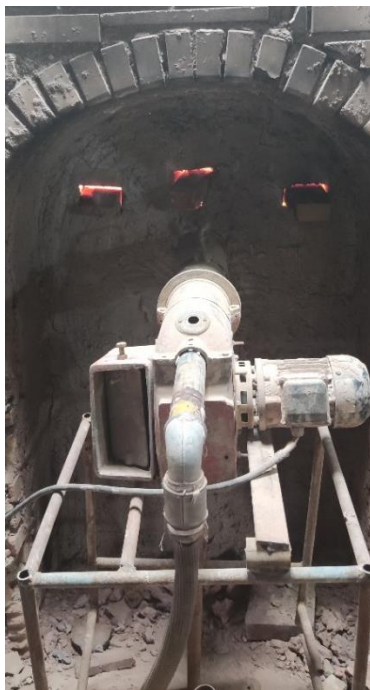
Figure.4.14. Gas injection through gas pipelines
