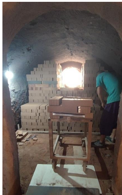
Figure 4.15. Stacking refractory bricks by labors in the kiln
