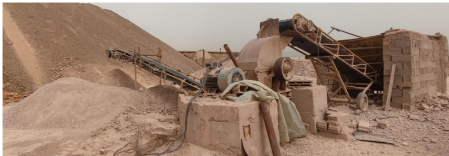
Figure 4.2. First Mill System to grind and crush the boulders into smaller pieces for the refractory brick
