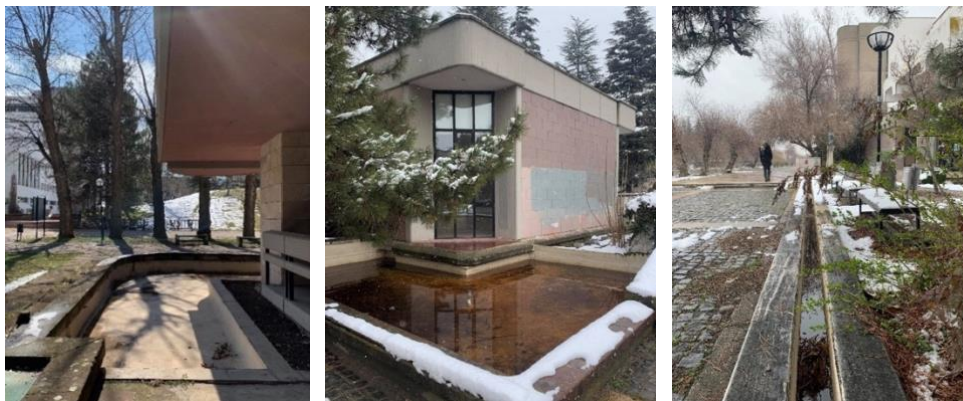
Figure 4.11: Main library building
