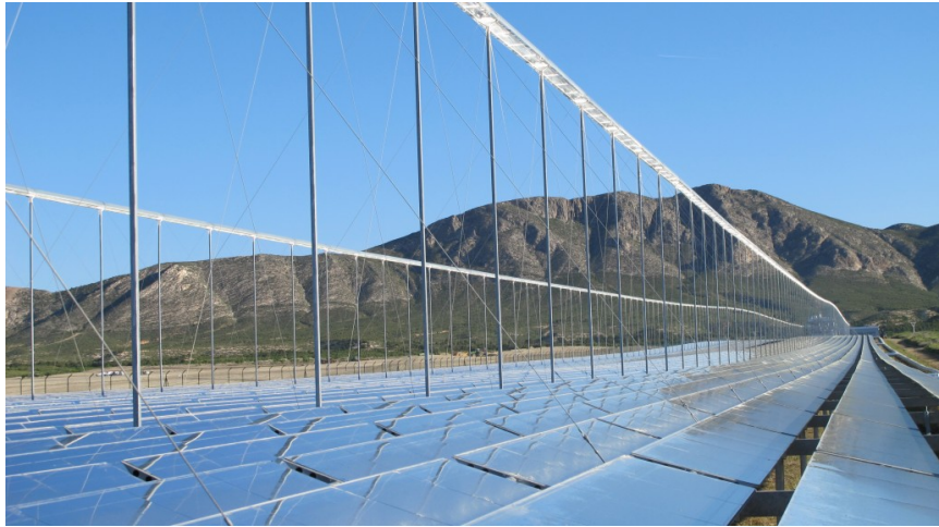
Figure 1.9: Linear Fresnel collector field at Puerto Errado 2 solar power plant [26].
