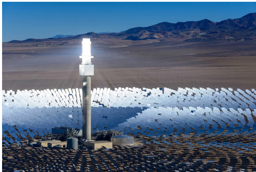
Figure 1.5: Crescent Dunes central receiver system solar power plant, Worland J. and Raab J. [21].
