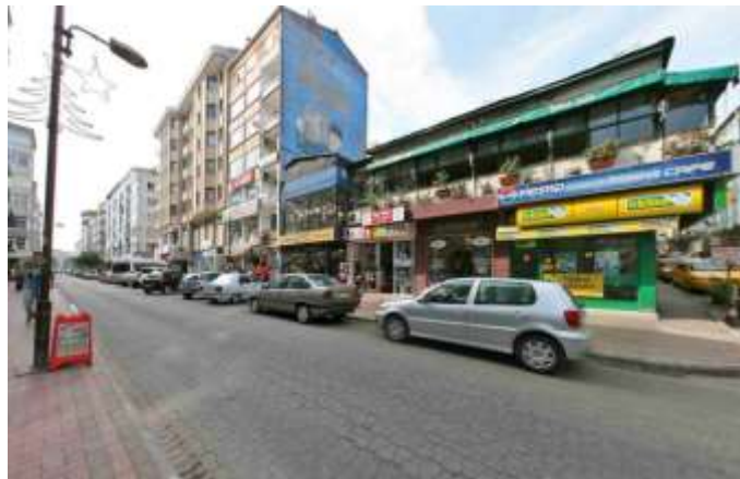
Figure 5.17. Building facades before the renovation (Samsun Metropolitan Municipality, 2019).
