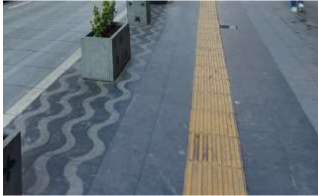
Figure 5.14. Surface covering in Çiftlik Street (Author's personal archive).
