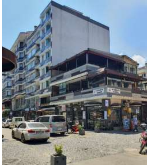
Figure 5.18. Building facades after the renovation (Author's personal archive).
