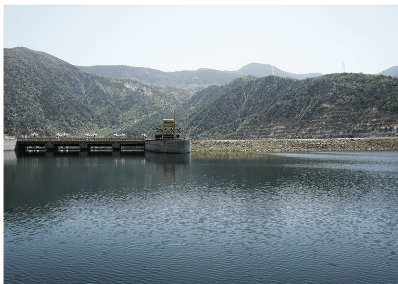
Figure 4.21 Oguzlar Dam. Photograph taken by the author, 2022.
