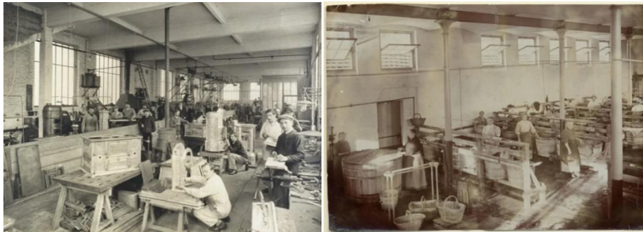
Figure 2.13 Interiors of the workshop and laundry room. Source: familistere.com
