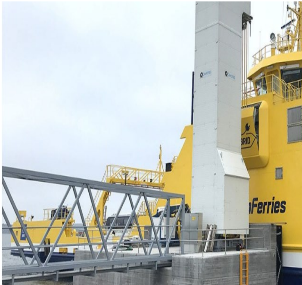
Figure 3.12. Tower-type chargers are ideal for charging Ro-Ro ferries in İzmir. Photo from [60].
